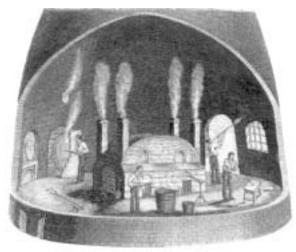
**Fig.5** Crown glass-making C.1860. Crown glass was made by blowing a bubble of glass, opening one end, and gradually widening it out until a large flat disc known as the 'crown' was formed. Small panes could then be cut from the crown.
