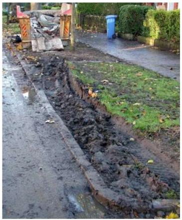
Figure 31 This ruinous damage to the verge was caused by a lorry delivering a skip
