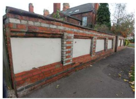
Figure 18 Original boundary wall with rendered, painted recesses (Salisbury St. and Park Ave.)
