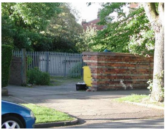
Figure 29 Original brick banded wall left in state of disrepair for many years – now demolished (Princes Ave. / Park Ave.)
