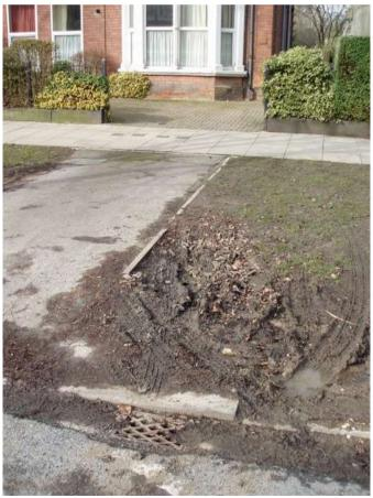
Figure 32 Damaged verge due to misuse of crossover
