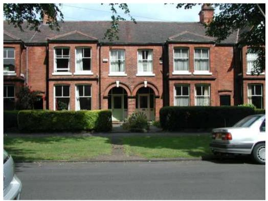
Figure 48 Traditional details make up a well-proportioned façade. Original open porches. (Westbourne Ave.)
