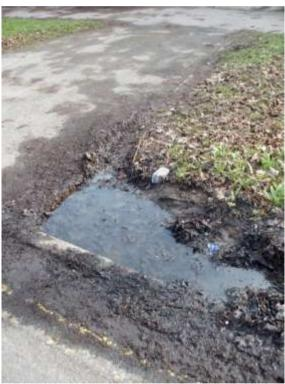
Figure 20 Damaged verge at a vehicular crossover
