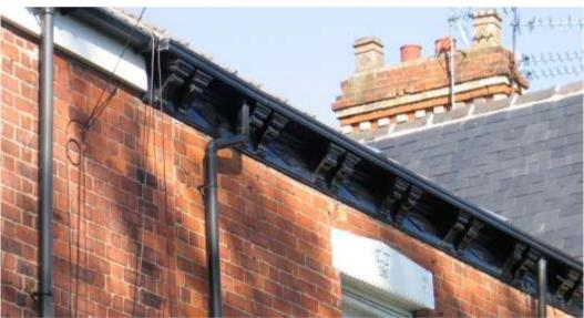
Figure 113 Modern PVCu fascia lacks the detailing and character of original timber fascia board (with diamond-shape relief and twin gutter blocks) and contrasts harshly with the original, creating discontinuity in the terrace (Westbourne Ave.)
