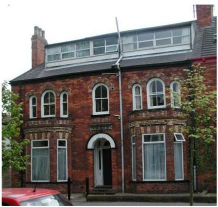
Figure 25 Loss of original character through installation of long block of modern dormer windows which overpowers the roofline; and replacement of Victorian sashes on ground floor with out-of-character large-paned windows, with small top-hung casements (Marlborough Ave.)
