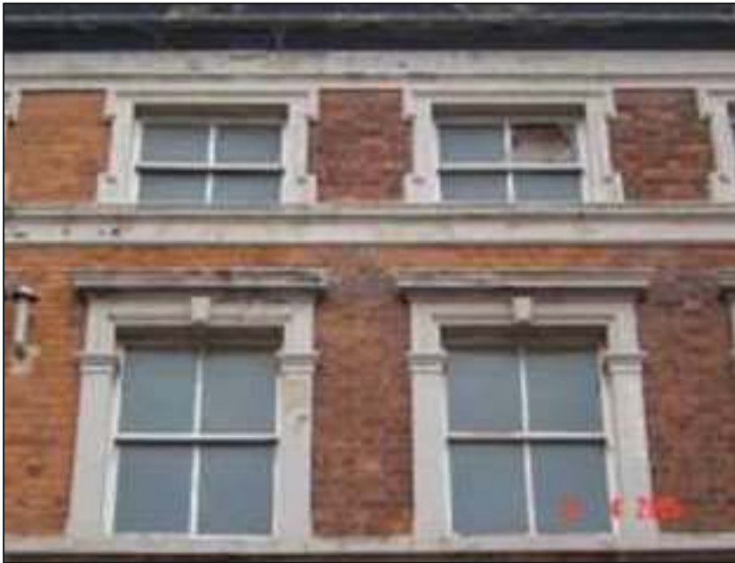
Figure 58: 2-over-2 timber sash windows
