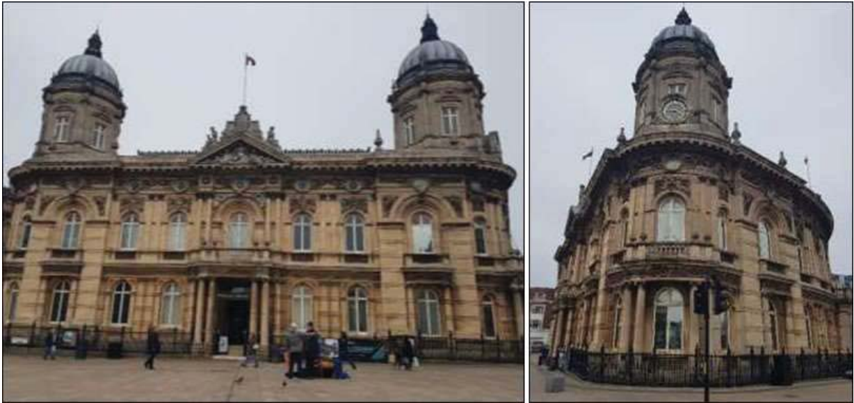
Figures 53 and 54: The former Dock Offices, now Hull Maritime Museum
