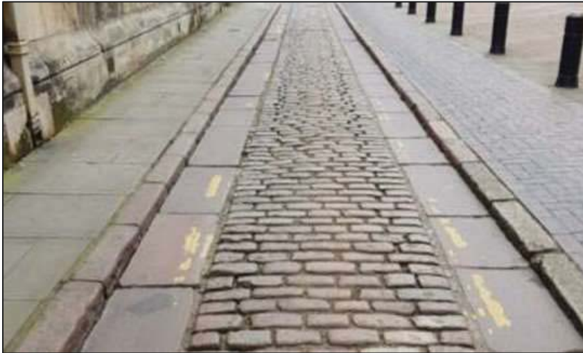
Figure 22: A photograph capturing some of the paving materials used in the Old Town (York stone paving; granite sets, gully stones and kerb stones; and modern brick block paving).
