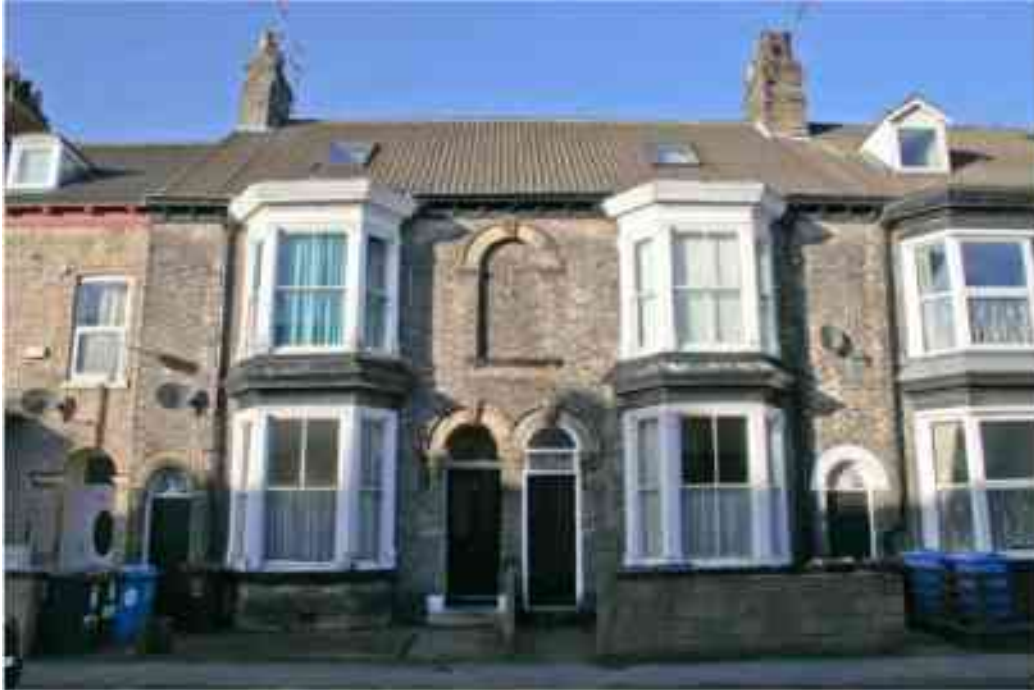
Figure 199 Nos. 6 & 8, Grove Street, front
