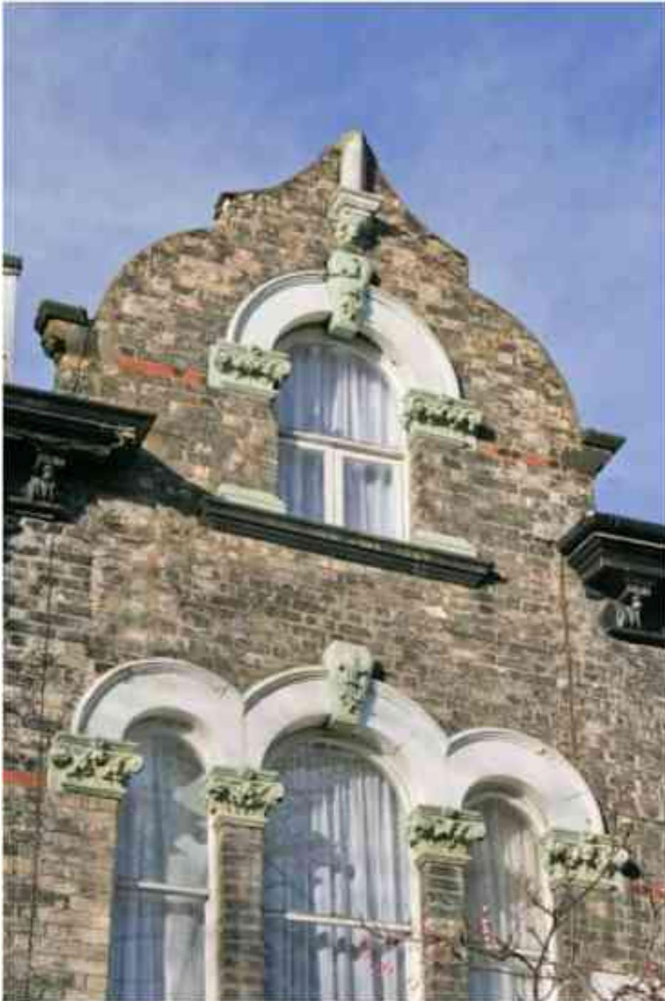
Figure 174 No. 10 Pearson Ave gable end
