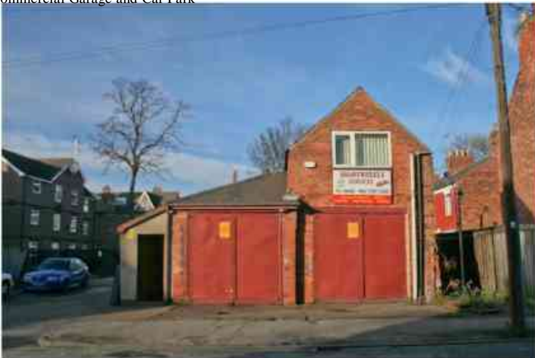
Figure 207 Commercial Garage front, Grove Street
