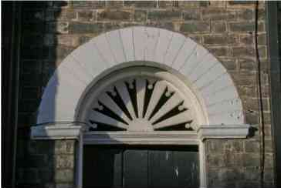
Figure 197 Nos. 4 & 6, Grove Street, passage detail
