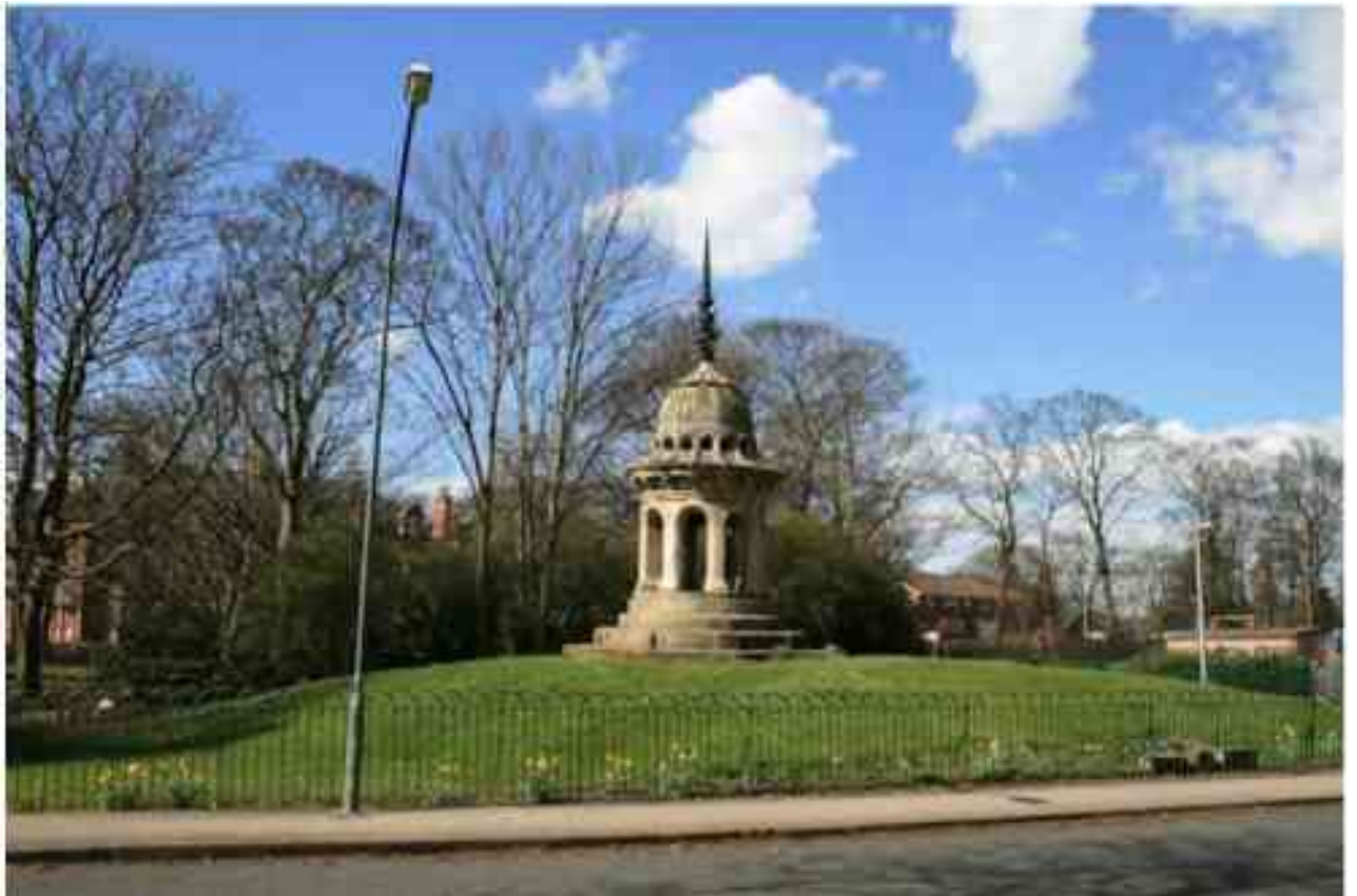
Figure 92 Cupola (prior to removal of bow-top fencing in 2013)
