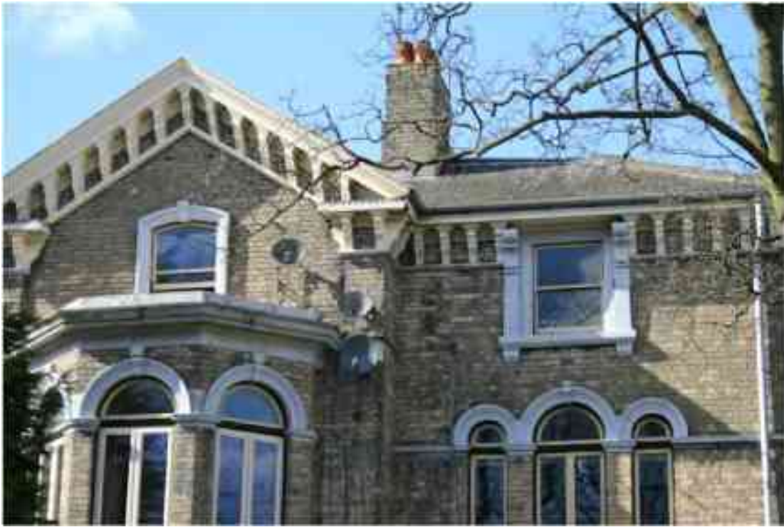
Figure 126 No. 56 front angle detail
