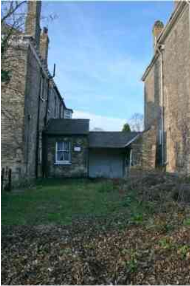
Figure 188 No. 20 Pearson Ave connecting corridor
