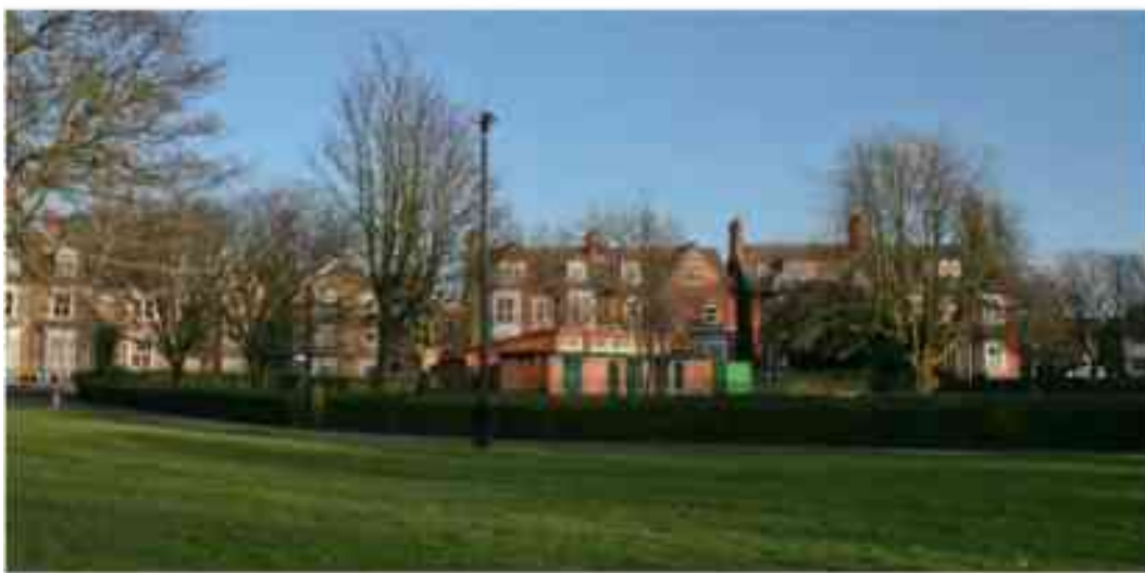
Figure 38 Bowling Pavilion view from west
