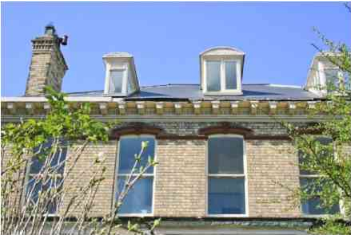
Figure 103 No. 43 top windows
