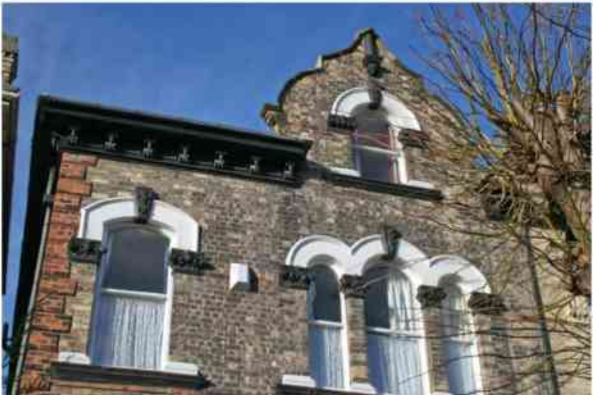
Figure 181 No. 18 Pearson Ave first floor
