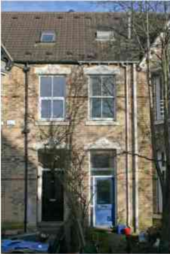
Figure 147 Nos. 64 & 65 front doors
