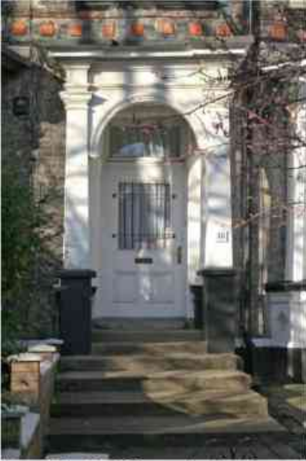
Figure 175 No.10 Pearson Ave front door
