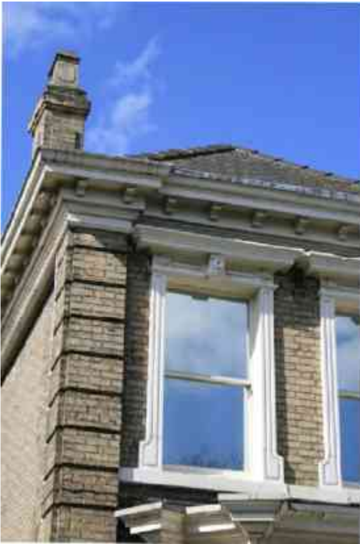
Figure 116 No. 50 first floor window and roof
