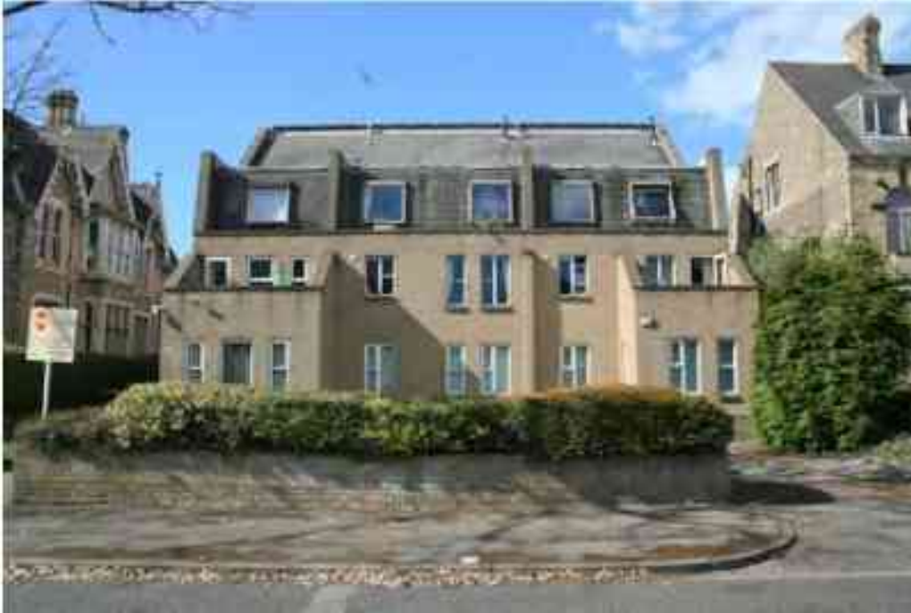
Figure 132 No. 59 - 70s flats - front
