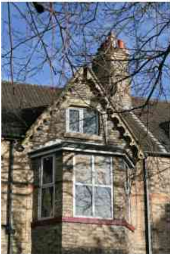
Figure 143 No. 63 gable detail
