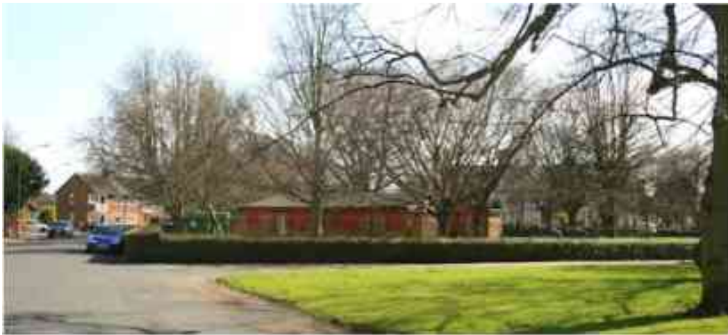
Figure 37 Bowling Pavilion view from north
