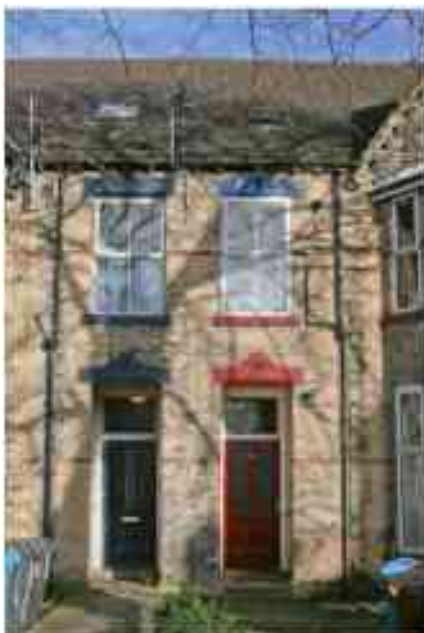
Figure 141 Nos. 62 & 63 front doors
