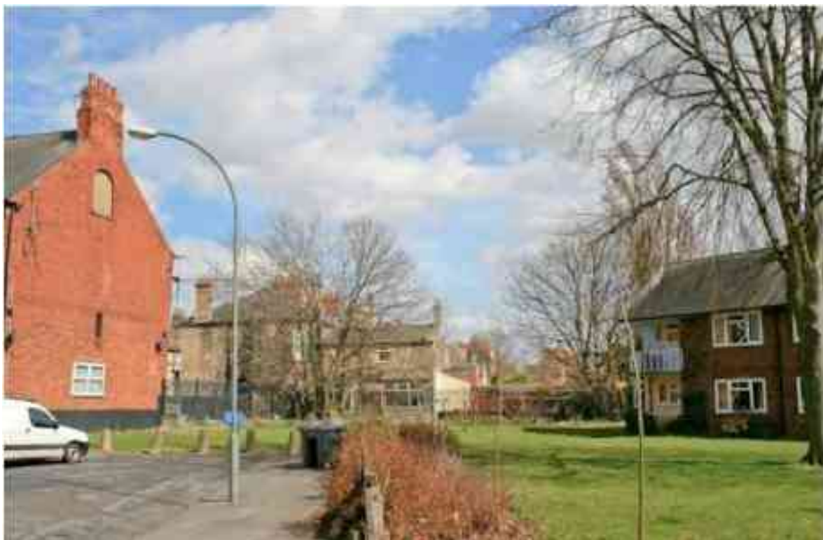
Figure 54 No. 9 side wall and start of Henson Villas
