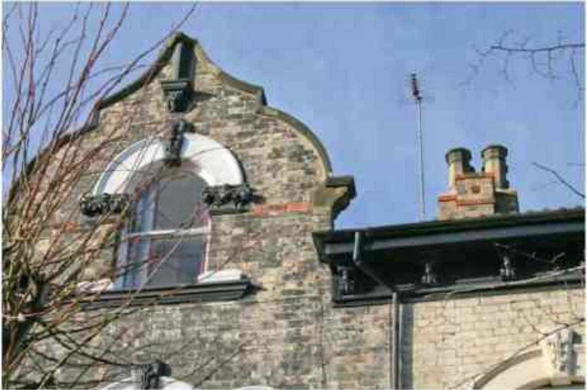
Figure 180 No. 18 Pearson Ave gable
