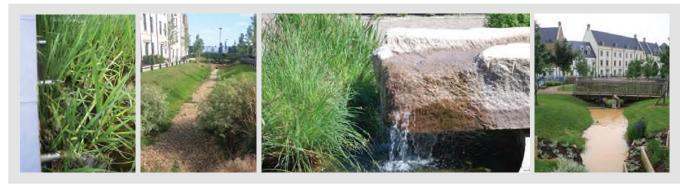
Site controls address run-off near source and include measures such as swales and permeable surfaces
