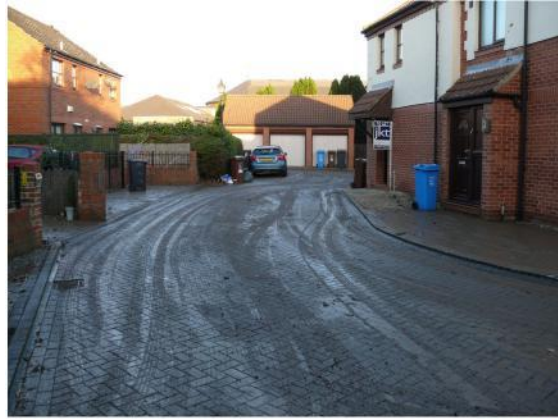
Evidence of flooding at the Anchorage
