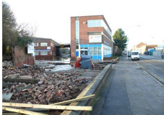
Wall destroyed by flood waters, English Street
