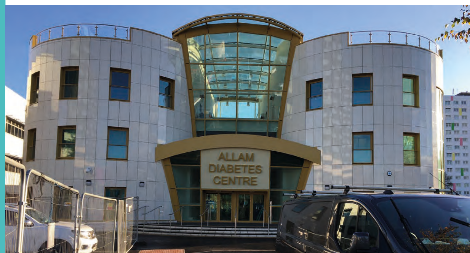
Figure 2.15: Site photograph of the Allam Diabetes Centre, designed by ACA.
