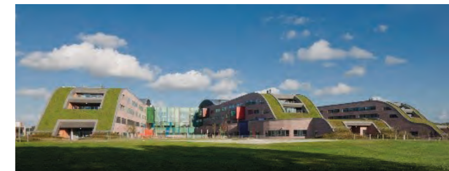
Figure 6.12: Example of Green Roof – Alder Hey Hospital
