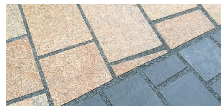
Figure 6.13: Example of Permeable Paving
