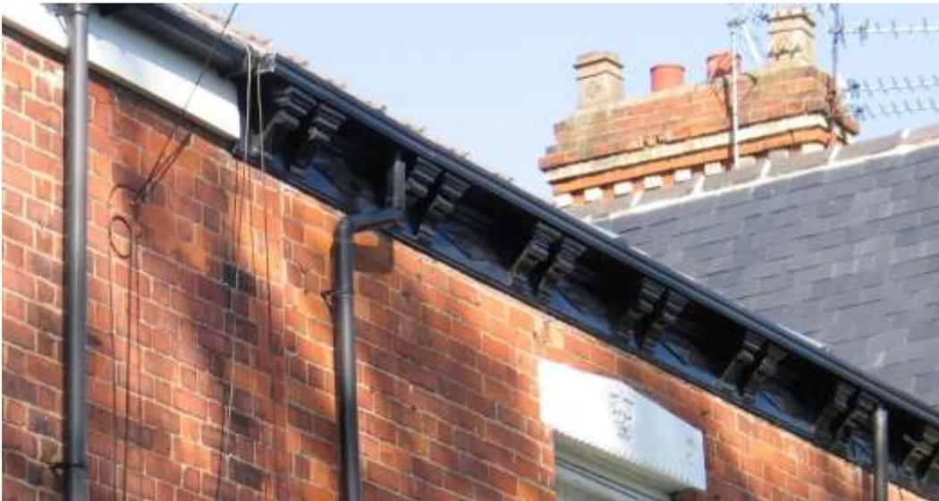
**Figure 113** Modern PVCu fascia lacks the detailing and character of original timber fascia board (with diamond-shape relief and twin gutter blocks) and contrasts harshly with the original, creating discontinuity in the terrace (Westbourne Ave.)
