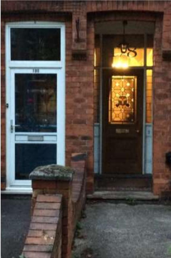
**Figure 99** Good example of a leaded light front door, with its house number featured in the overlight: in stark contrast to the adjacent out-of-character storm door (Victoria Ave.)
