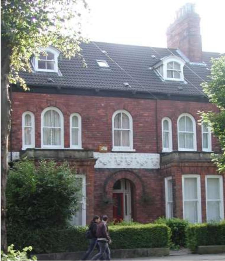
**Figure 58** Victorian terrace dating from the early years of The Avenues development. Unfortunately, the original roof slates have been replaced with modern concrete tiles. (Westbourne Ave.)
