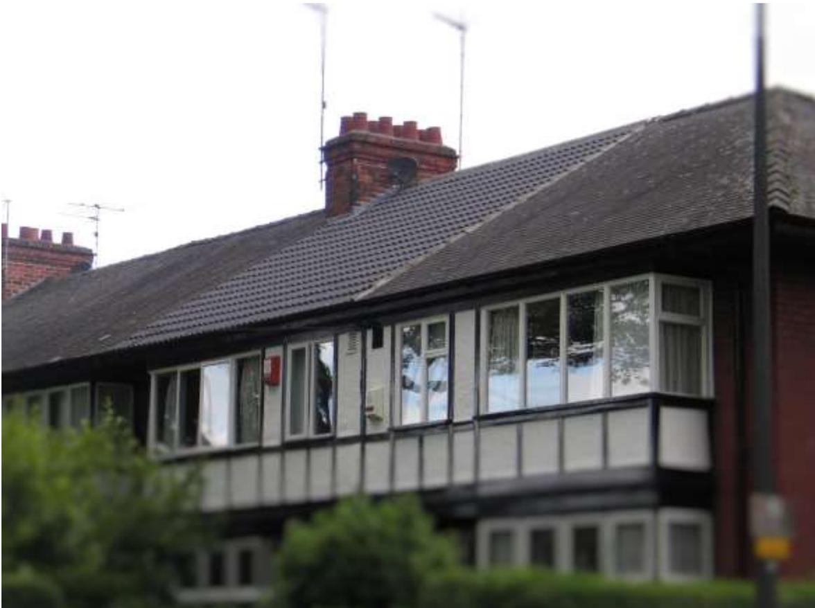
**Figure 28** The original harmony of these roofs is destroyed by the replacement of slates with tiles of different material, design and thickness, brutally interrupting the continuous slate roof across this terrace of houses (Westbourne Ave.)
