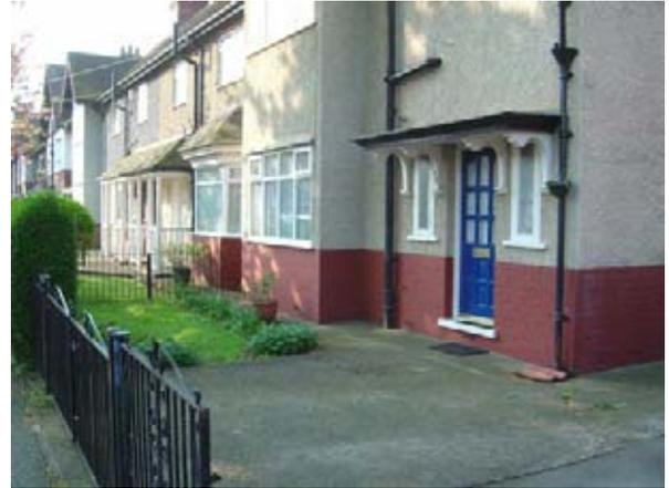
**Photo 13: Brick & roughcast terrace-of-4 featuring square and cant bay windows, canopies and projecting open porches.**
