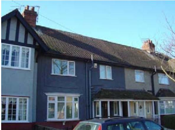
**Photo 21:** Unsympathetic modern bow window in place of an original canted bay.
