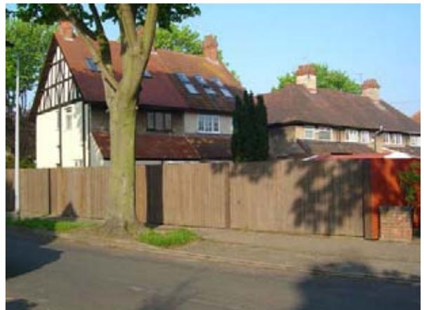
**Photo 30: Unsympathetic (non- conservation type) rooflights.**
