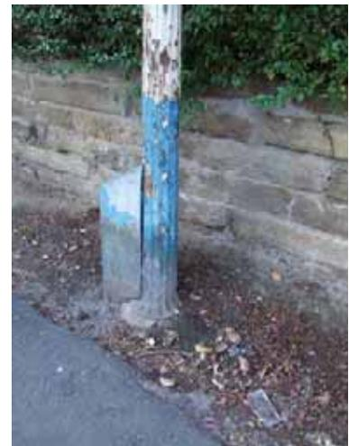
Figure 20.2 gas lamp standard with fluted base.
