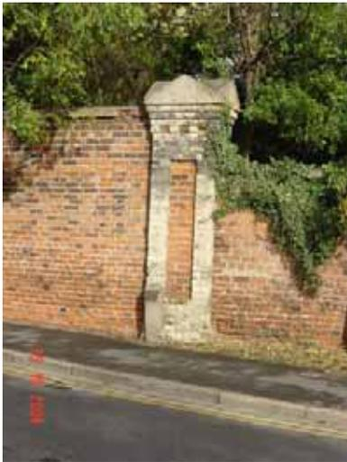
Figure 12.2 Polychrome pier in boundary wall of Beech Lawn and the Elms.
