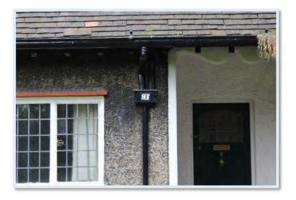
Figure 50 - Timber gutters and original hoppers at 6 The Oval.
