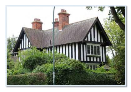
Figure 57 - Timber Panelling & Barge Boards at 71 Village Road.
