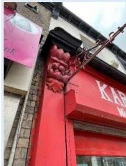
Figure 53 - Retained console bracket to No 157 Spring Bank (Author, 2023)
