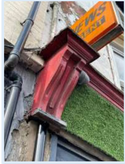
Figure 47 - Retained console bracket to No 21 Spring Bank (Author, 2023)
