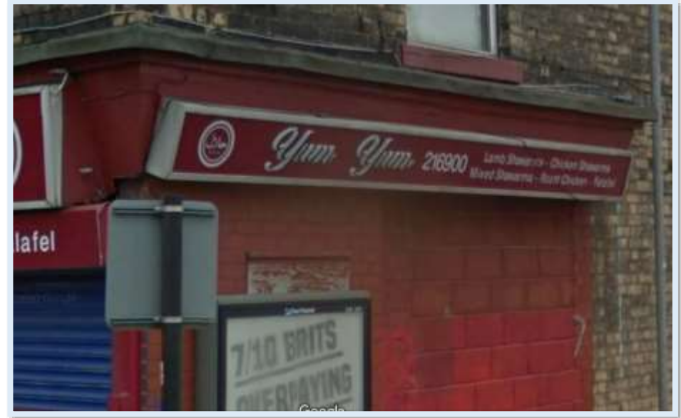
Figure 41 - Retained cornice detail to 141 Spring Bank (Author, 2023)
