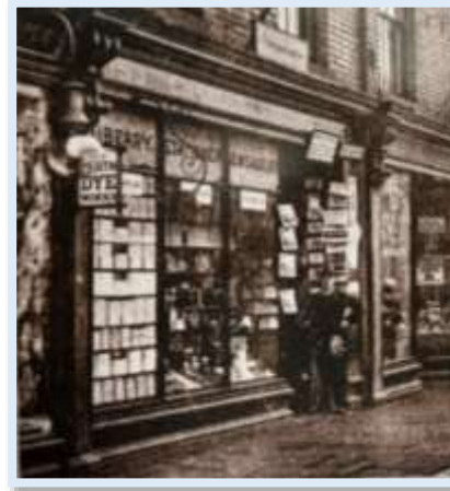
Figure 82 - Historical photograph from C1905 showing the carved stone stall riser (Gibson, Hull Then and Now, Volume 1, 2008)
