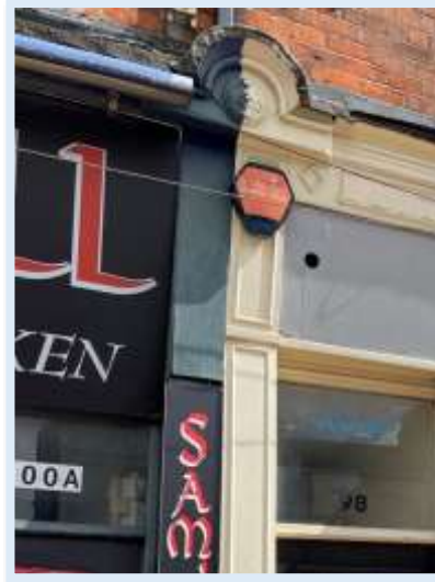
Figure 58 -Retained console head to No 94/98 Spring Bank (Author, 2023)
