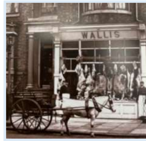
Figure 64 - Historical photograph from 1905 showing the south side of Spring Bank and the decorative corbels to No 109 (Gibson, Hull Then and Now, Volume 1, 2008)
