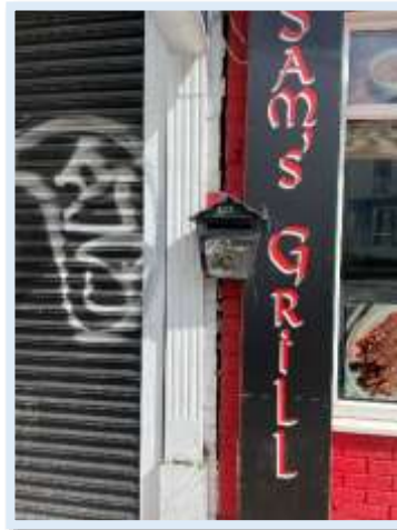
Figure 44 - No 104 Spring Bank showing the retained pilaster detail (Author, 2023)
