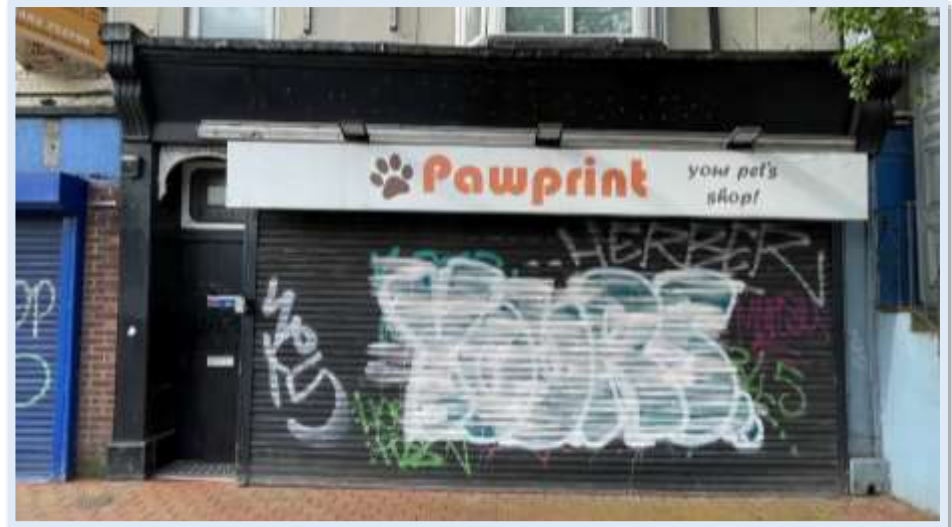
Figure 43 - No 45 Spring Bank showing the retained pilasters and console brackets dating from the late 1800's. (Author, 2023)
