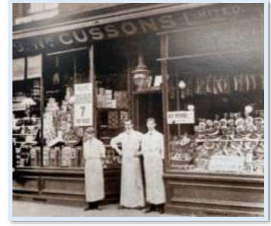
Figure 81 - Historic photograph of Spring from C1950 showing the timber panelled stall riser. (Gibson, Hull Then and Now, Volume 1, 2008)
