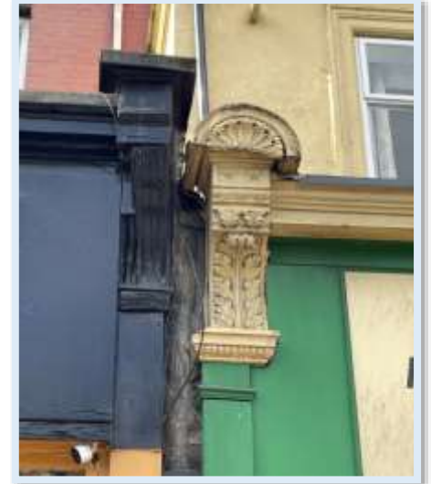
Figure 48 - Retained console brackets to No 45 and 47 Spring Bank (Author, 2023)
