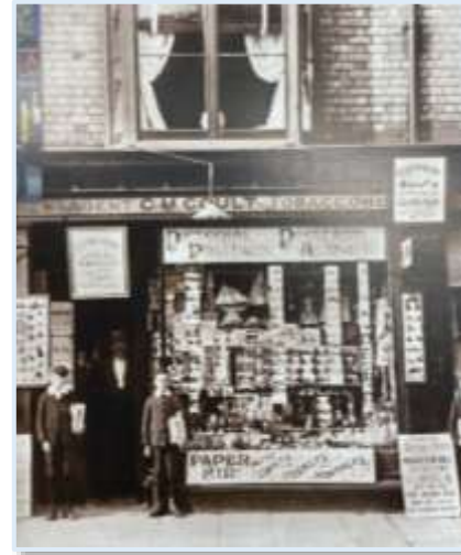
Figure 84 -Historical photograph from 1904/1905 showing the use of transom lights shopfronts on Spring Bank (Gibson, Hull Then and Now, Volume 1, 2008)
