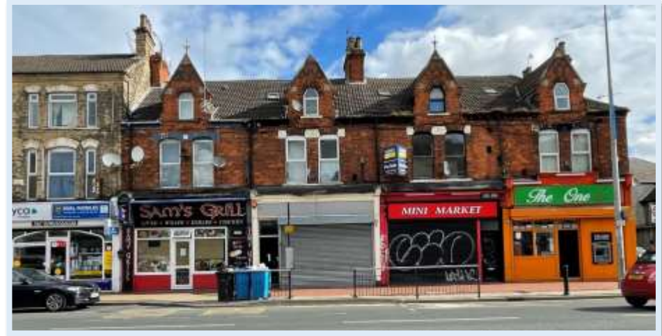
Figure 65 - Examples of the extent of metal shutter installation to the shopfronts along Spring Bank (Author, 2023)
