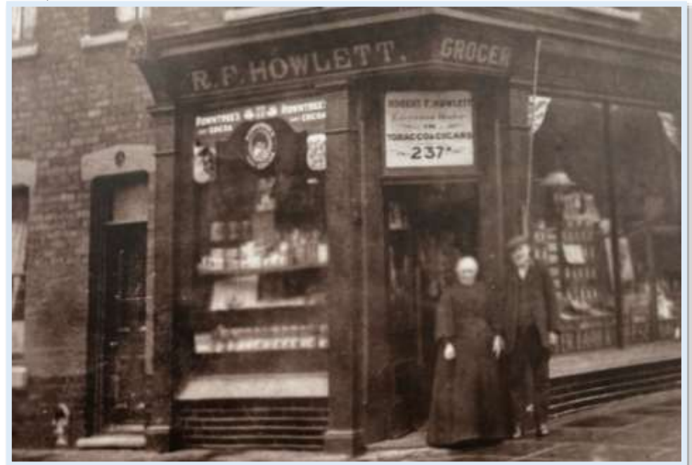
Figure 83 - Historic photograph from c1905 showing a brick stall riser. (Gibson, Hull Then and Now, Volume 1, 2008)
