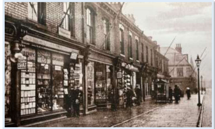
Figure 63 - Historical photograph from 1905 showing the south side of Spring Bank and the decorative corbels from No 153- 159 (Gibson, Hull Then and Now, Volume 1, 2008)
