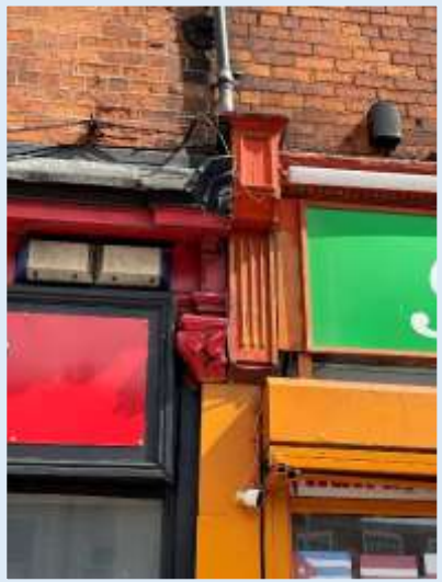
Figure 61 -Retained console bracket to No 98 Spring Bank (Author, 2023)
