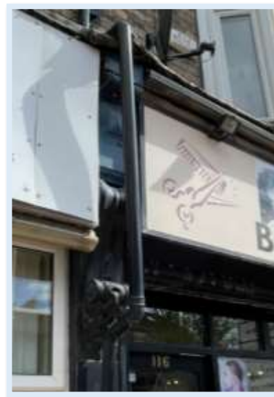
Figure 57 -Retained console bracket to No 118 Spring Bank (Author, 2023)
