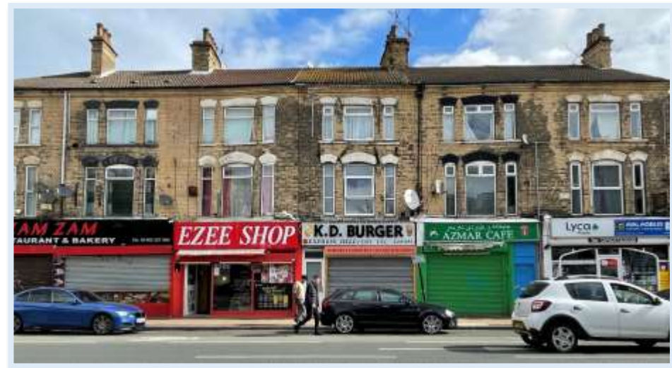
Figure 66 Examples of the extent of metal shutter installation to the shopfronts along Spring Bank (Author, 2023)
