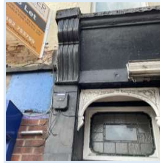
Figure 42 - Retained cornice detail to 45 Spring Bank (Author, 2023)
