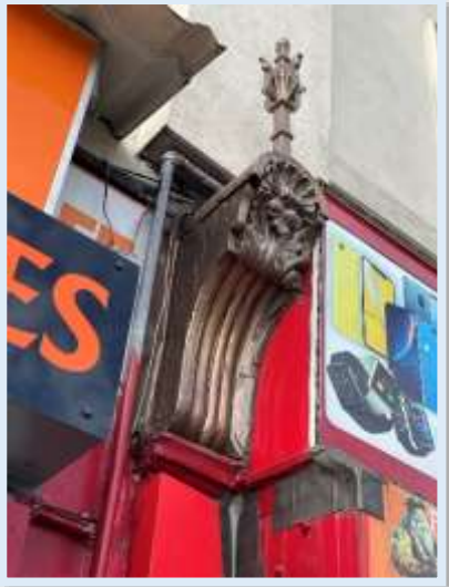
Figure 49 - Retained console bracket to No 19 Spring Bank (Author, 2023)
