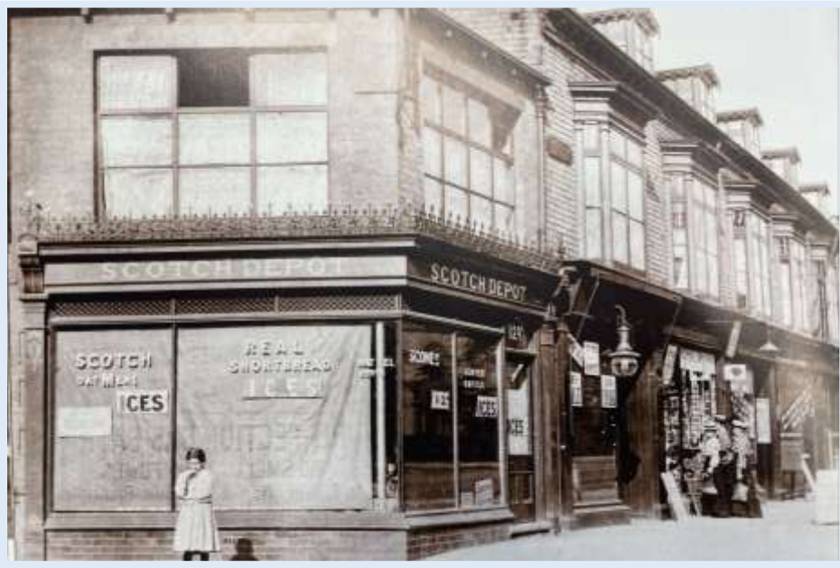
Figure 75 - Historical photograph from 1904 showing 129a and 129 adjacent on the south side of Spring Bank where the provision of an awning to the top of the fascia can be seen. (Gibson, Hull Then and Now, Volume 3, 2012)
