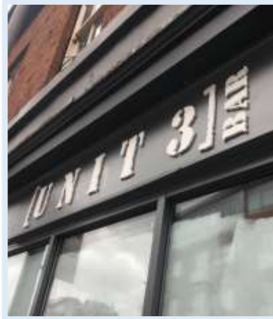
Figure 39 -Cut out letters on a traditional fascia can provide a more modern solution (SIGRAMCR., n.d.)
