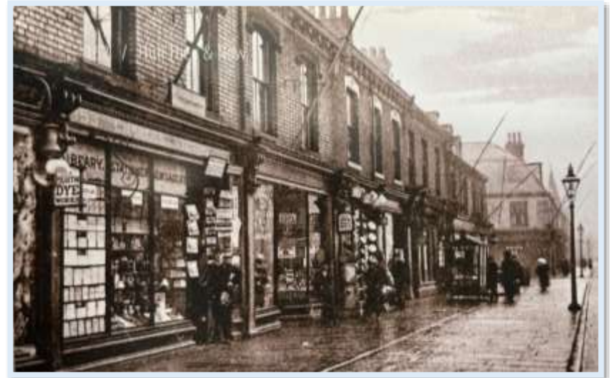
Figure 12 - Historical photograph from C1905 showing the styles of shopfronts installed on Spring Bank (Gibson, Hull Then and Now, Volume 1, 2008)
