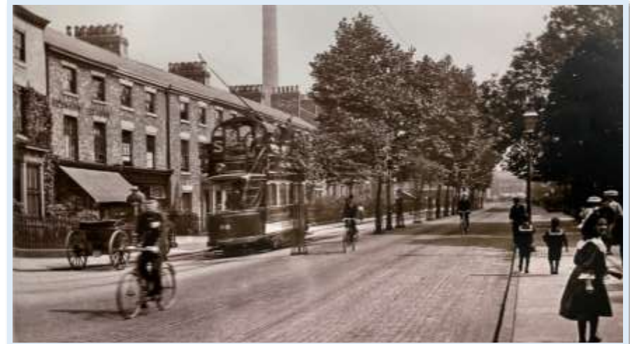
Figure 76 - Historical photograph from 1905 showing Brunswick Terrace to the north side of Spring Bank and the awning/blind to the Library. (Gibson, Hull Then and Now, Volume 1, 2008)
