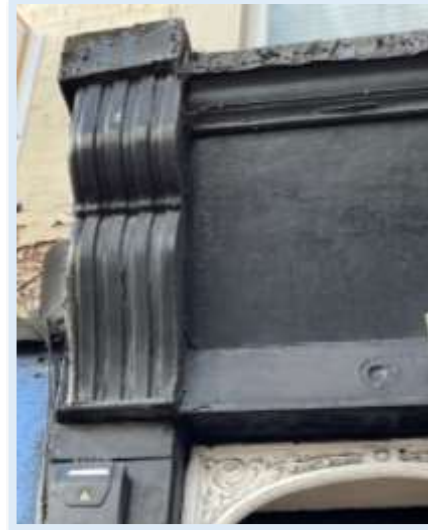
Figure 46 - Retained console bracket to No 21 Spring Bank (Author, 2023)
