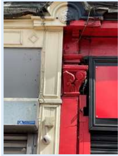
Figure 59 - Retained console bracket to No 96/98 Spring Bank (Author, 2023)
