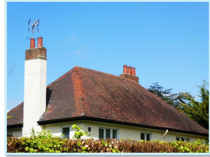
Figure 17 Hipped roof and clay tiles at No.90.
