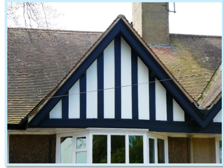
Figure 26 Close stud 'Mock' panelling.
