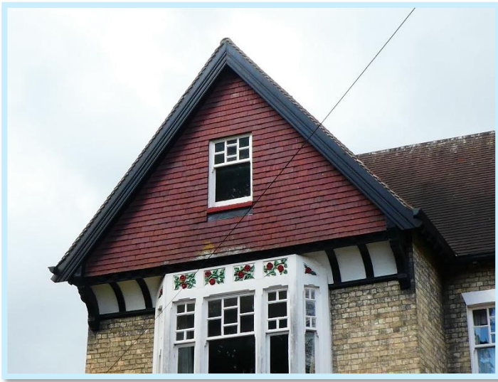
Figure 25 Tile cladding, decorative glazing, and plasterwork at No.45.
