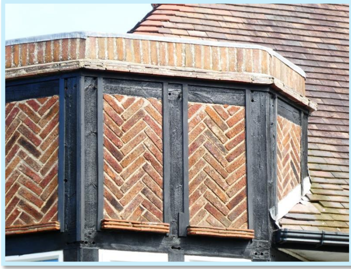
Figure 24 - Herringbone Brickwork at No.45.
