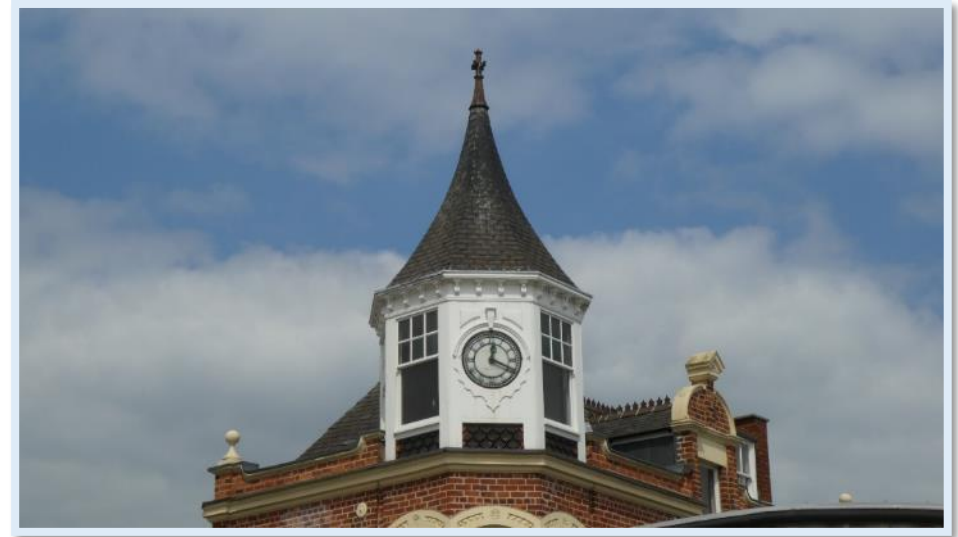
Figure 138 The clock tower at Pendrill House (Local Listed)
