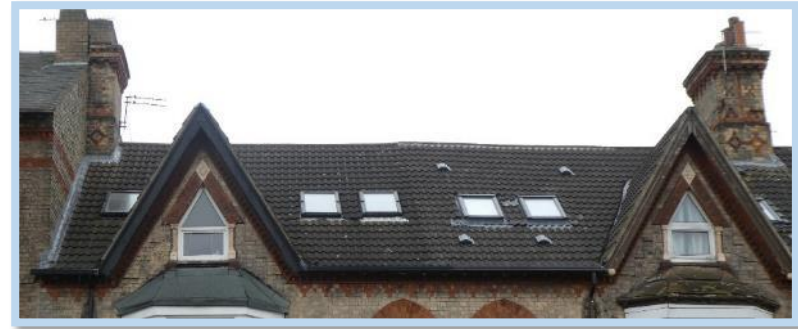
Figure 133 Cluttered roof profile at Nos.96-8
