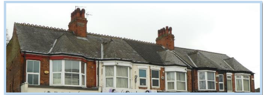
Figure 134 Nos.500-8 - Bay windows and cresting tiles.
