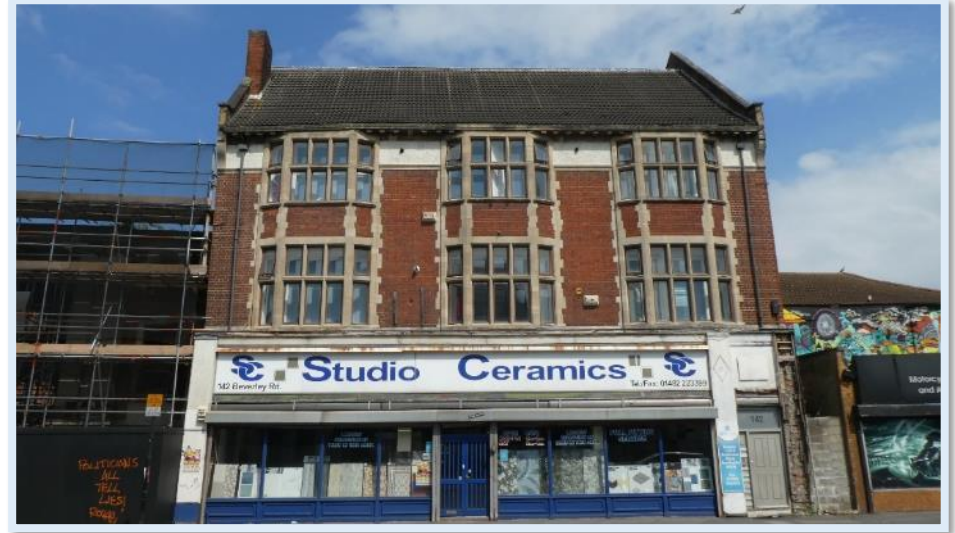
Figure 87 No.142 - Ground floor shop front does not match upper floors.
