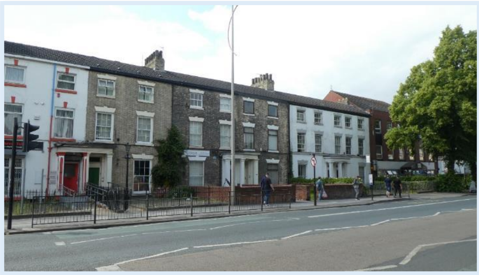
Figure 43 Nos.27-35 'Scarborough Terrace'
