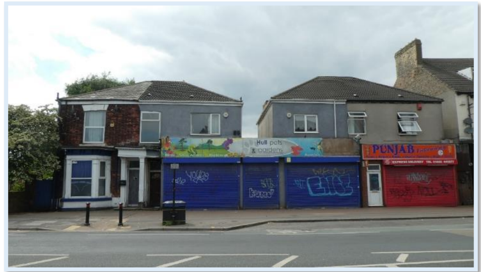
Figure 88 Nos.201-207 - Poor quality shop front additions.
