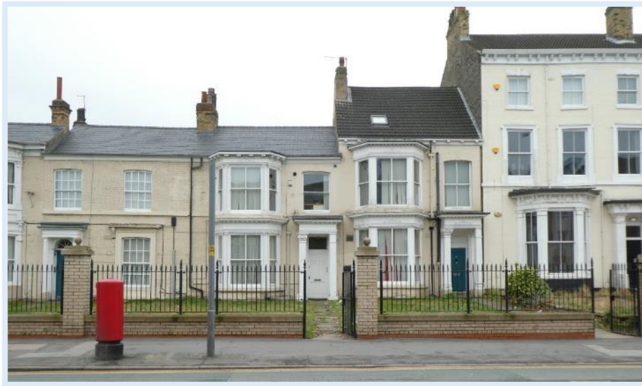
Figure 210 Nos.85-91 - Positive retention of historic joinery details and re-instated boundaries.
