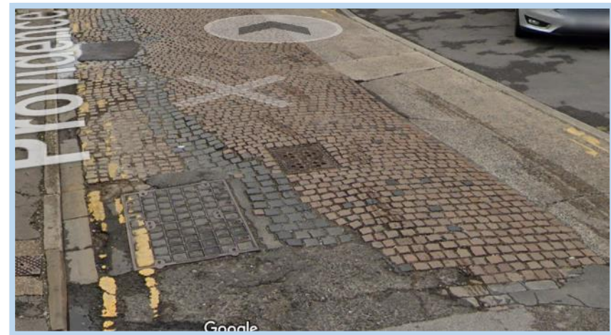
Figure 194 Historic setts in Providence Row (Google images)
