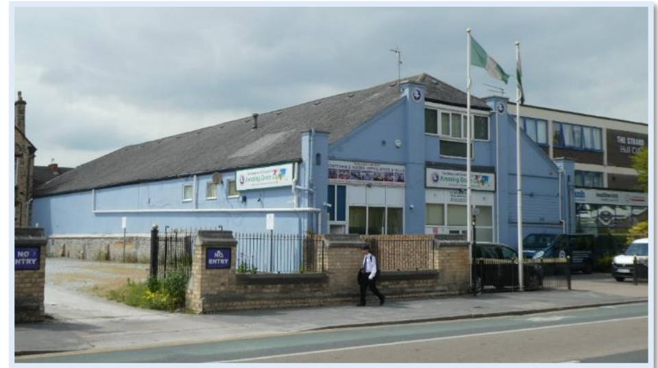
Figure 107 Lat 19th century former Warehouse, No.73.
