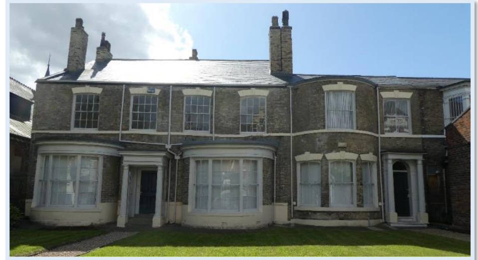
Figure 117 Multiple light and later 2/2 replacements at Nos. 53 and 55.
