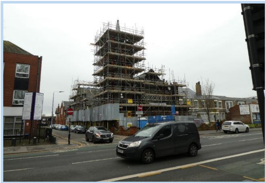
Figure 109 Trafalgar Street Church (works in progress at time of survey)
