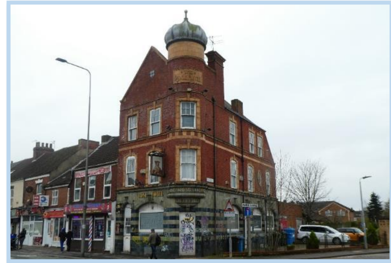
Figure 137 Decorative roof profile at the Rose Hotel (Local Listed)
