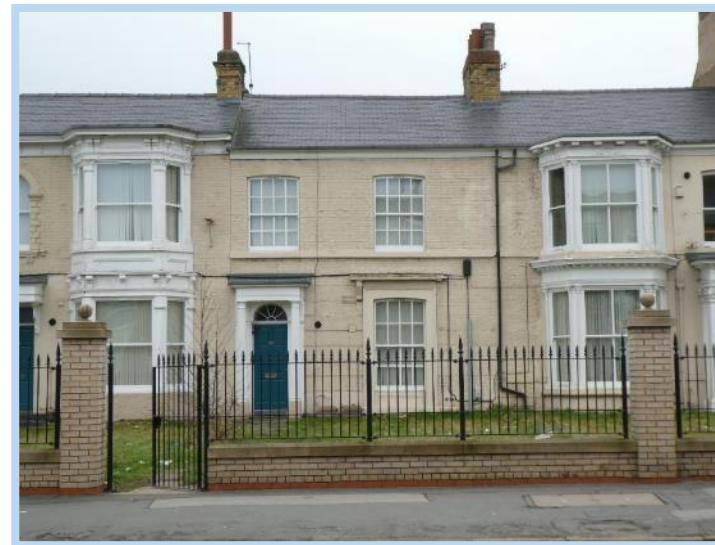
Figure 186 restored boundary treatments at No.89
