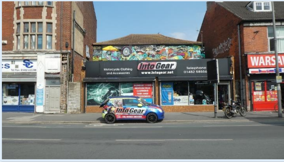
Figure 93 Poor quality ground floor frontages at No.140
