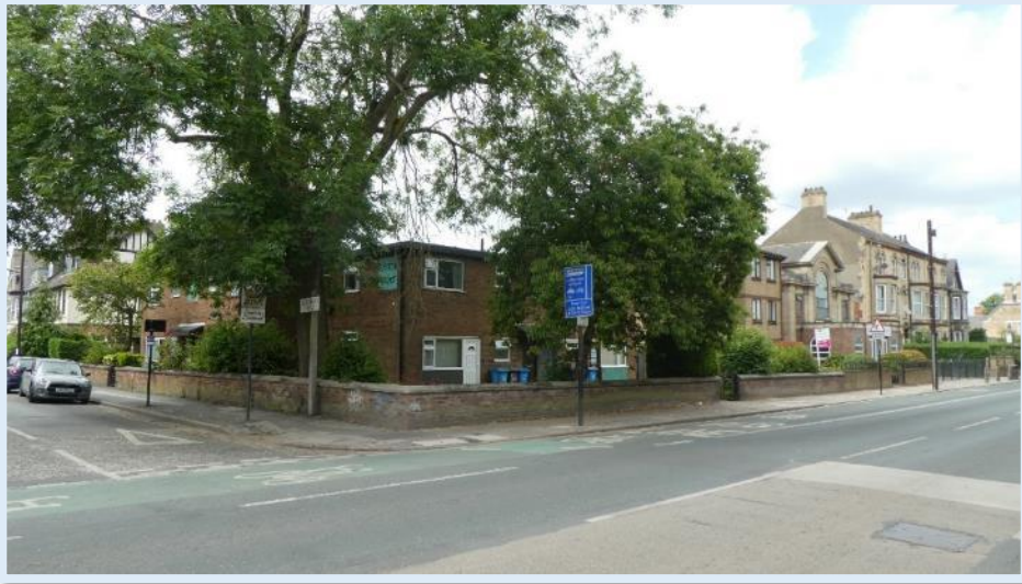
Figure 54 Easton Court and 381 Beverley Road
