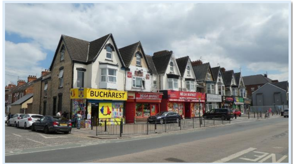
Figure 96 - Negative quality advertising & shops. Showing No.416 after works.
