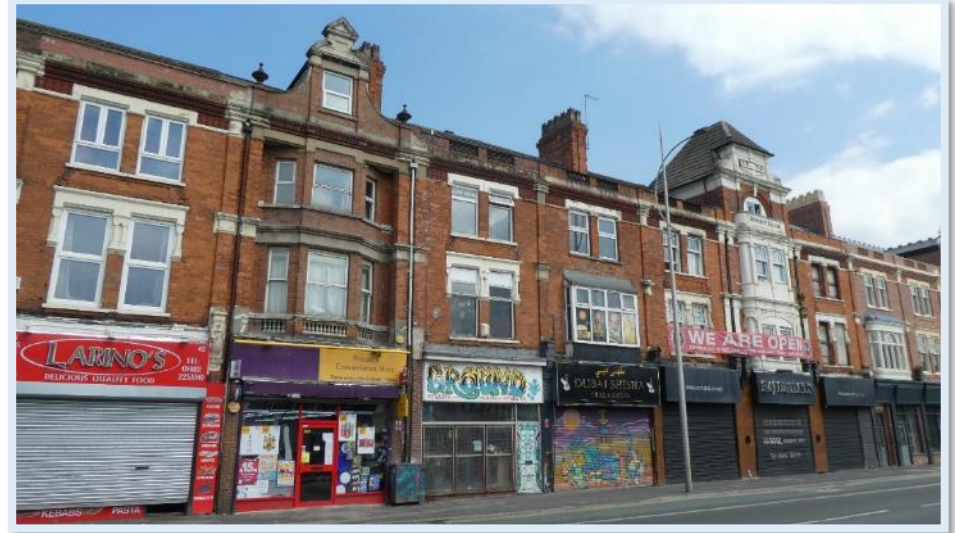
Figure 95 Brunswick Arcade - Negative quality shop fronts & advertising.
