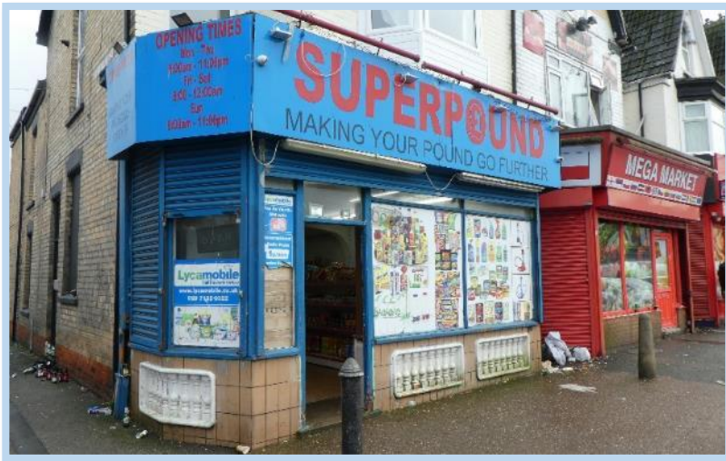
Figure 86 Nos. 414 and 416 - The prior retains a historic stall riser, but the shop fronts are of a poor-quality (showing condition before alteration in c.June 2024).
