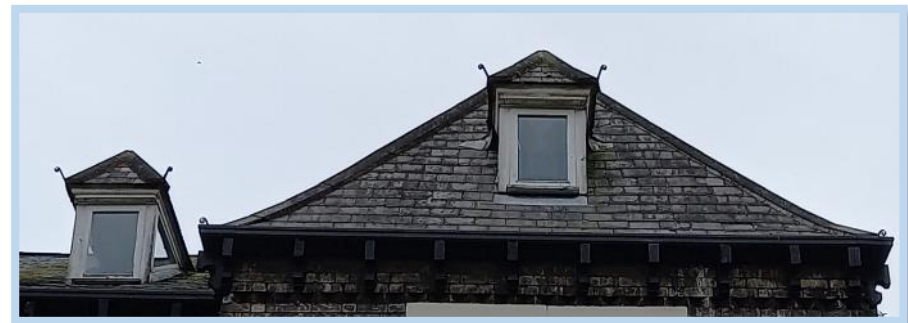
Figure 132 - Traditional types of dormer at No.265
