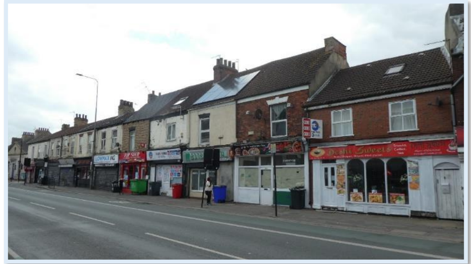
Figure 83 Negative quality shop fronts in Zone 2.
