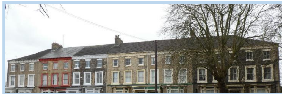
Figure 127 Nos 72-84 (Grade II) - Mid-19th century roof without dormers. Only one section retains traditional slates.
