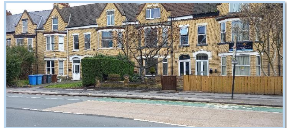
Figure 182 Nos. 352-348 - Open, restored and timber boundaries - a negative example.
