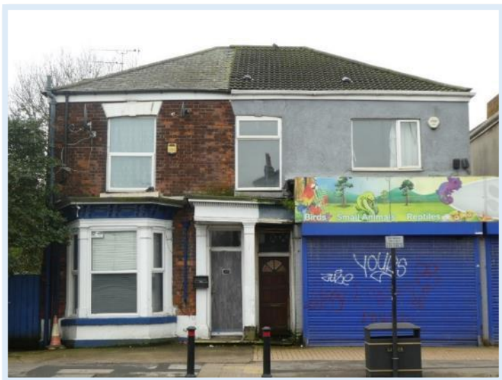
Figure 208 Potential to restore a residential façade and remove a poor-quality shop frontage at Nos.201-203
