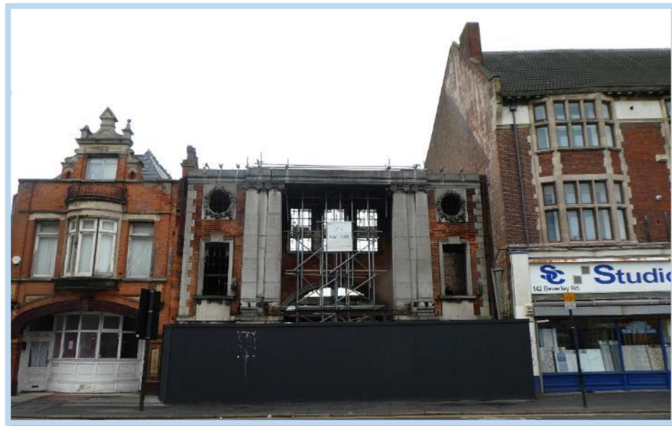
Figure 106 National Picture Theatre (Grade II) and Swan Inn (Locally Listed)
