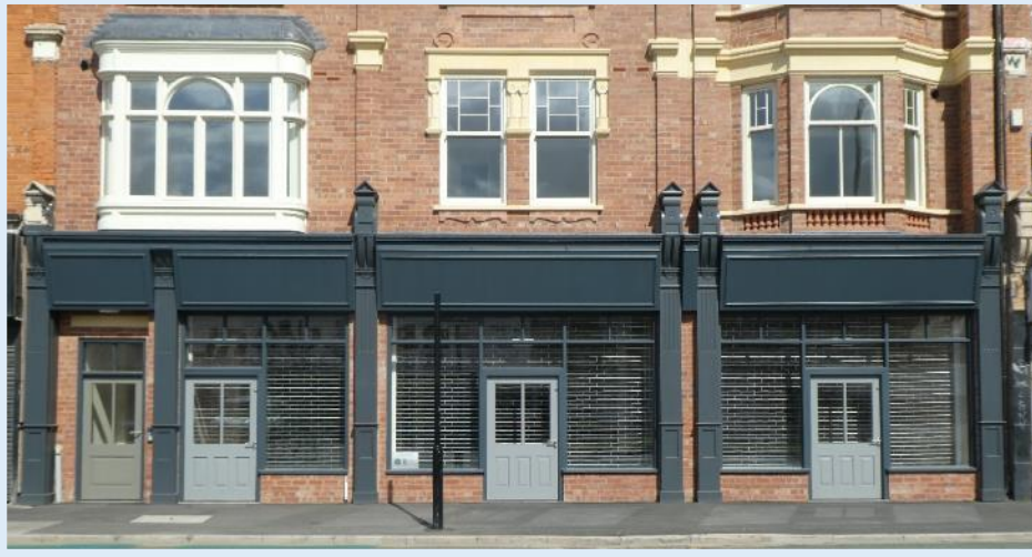
Figure 74 No.52-52a - THS shop front restoration, which incorporates the historic columns on the Brunswick Arcade.
