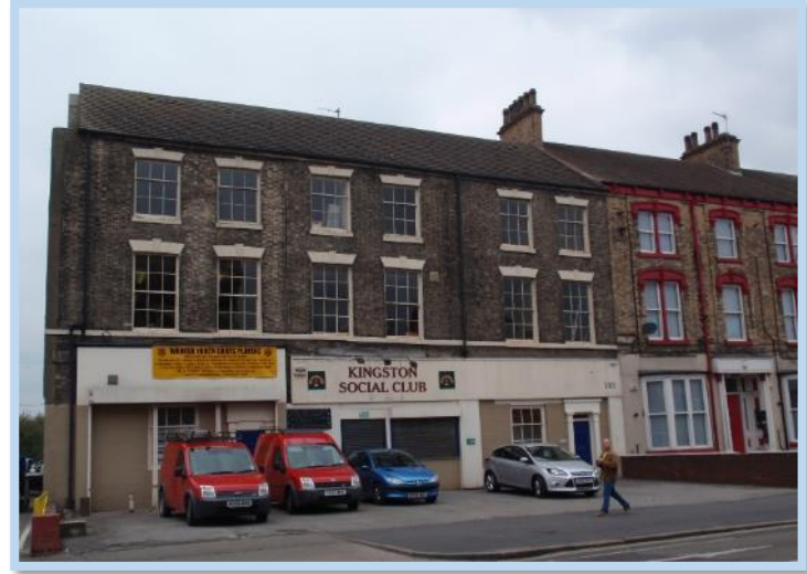
Figure 10 - Nos. 129-31 before restoration.
