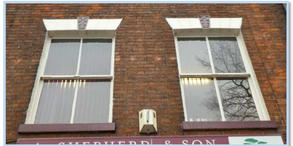
Figure 118 2/2 timber sliding sash windows at No.48
