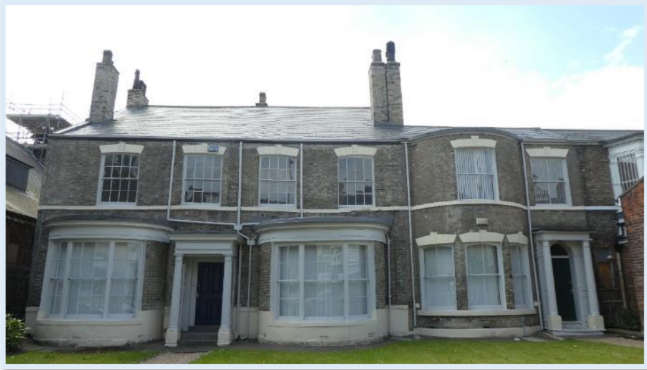
Figure 42 Nos.53 & 55 - 'York Terrace'
