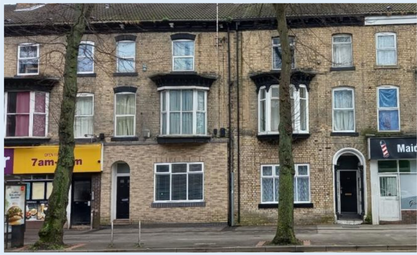
Figure 207 Nos. 213 & 314 Ground floor re-instatements without architectural decoration.
