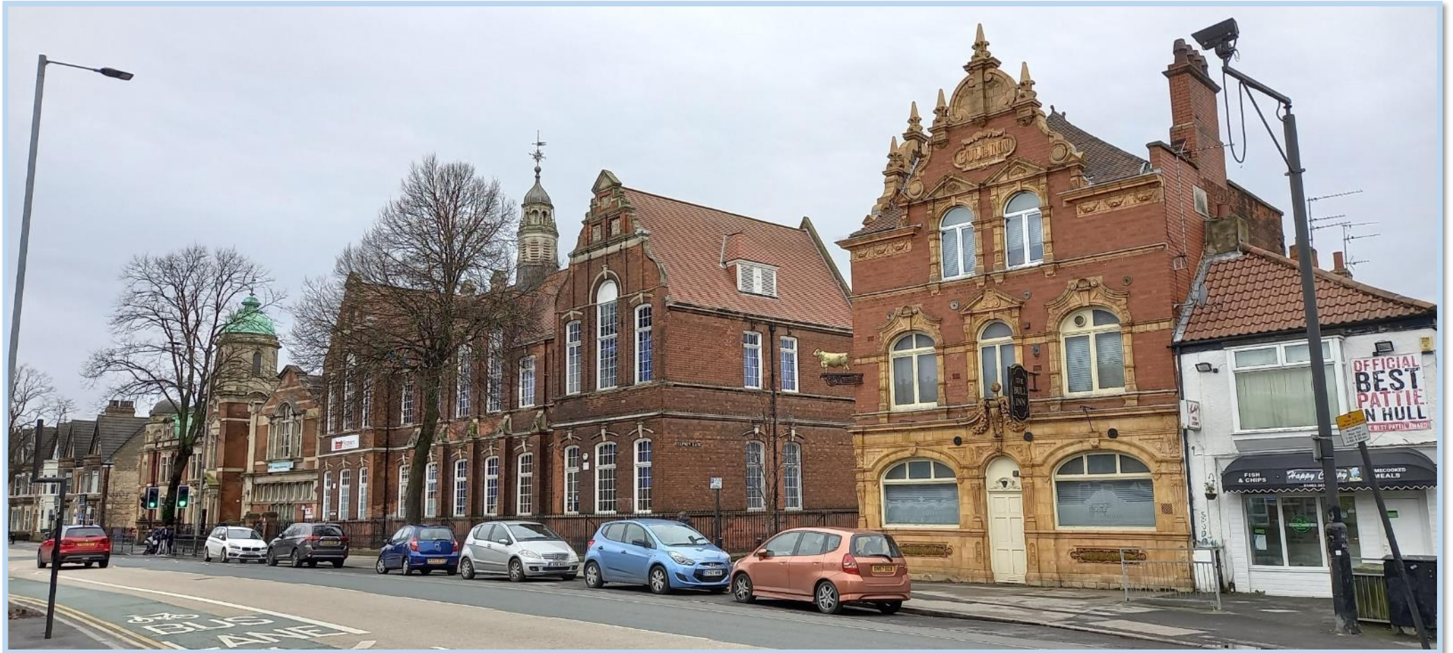
Figure 147 Important grouping of 'Key' - Bull Hotel, School & Baths – all listed Grade II.
