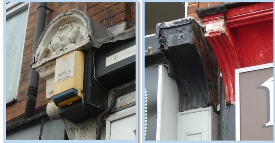
Figure 78 Elements of No.215 & 470 & 472, with columns replaced but capitals retained.
