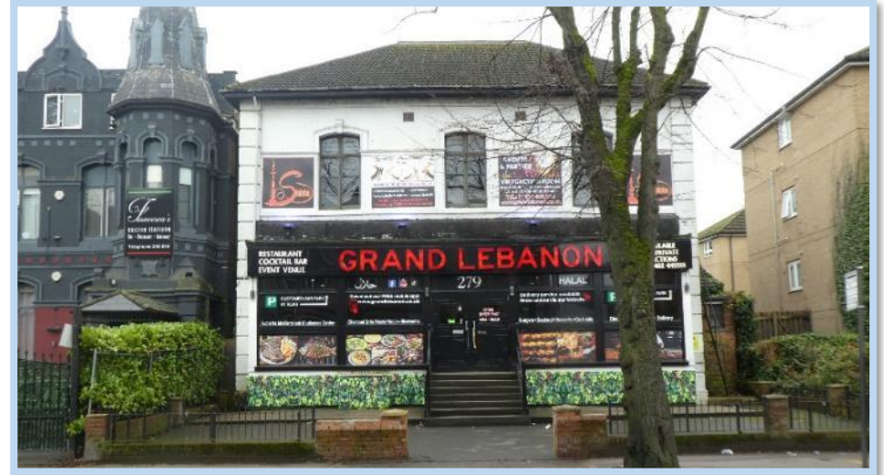
Figure 115 No.279 - Negative example of commercial frontage within Zone 3.
