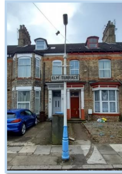
Figure 193 c.1950s lamp standard at Elm Terrace
