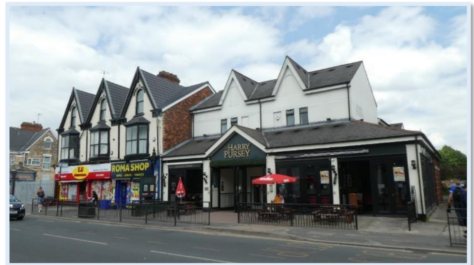
Figure 116 - Extension to No.386 Beverley Road.
