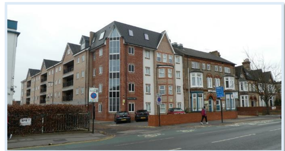
Figure 206 Consideration should be given to ridge lines and heights of side streets.
