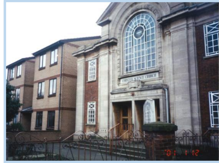
Figure 111 No.383 before extension.
