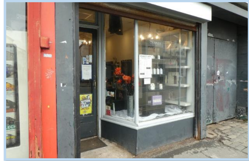
Figure 69 No.222 - Retained timber shop window & lobby, but with roller shutters.
