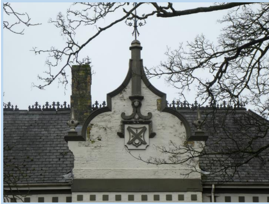
Figure 136 Shaped gable and cresting tiles at the Dorchester Hotel (Local Listed)
