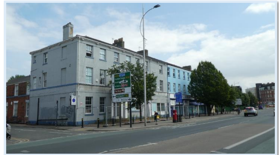
Figure 15 Nos.32-43 Beverley Road
