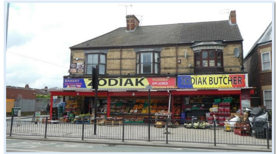
Figure 90 Canopy at 359 Beverley Road (Pending Enforcement at time of survey)
