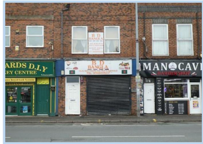
Figure 169 No positive feature retained at No. 178
