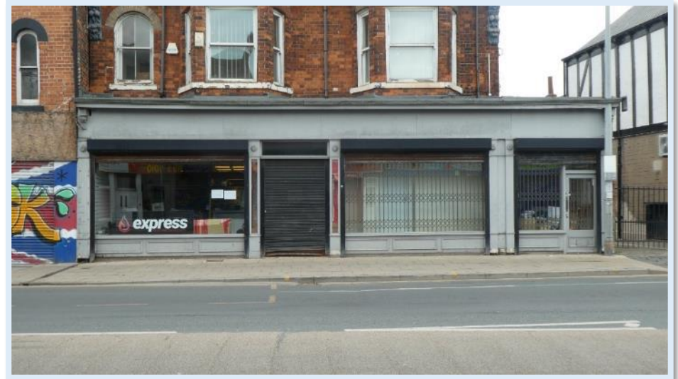
Figure 70 - No.206 - Positive quality timber shop front addition.
