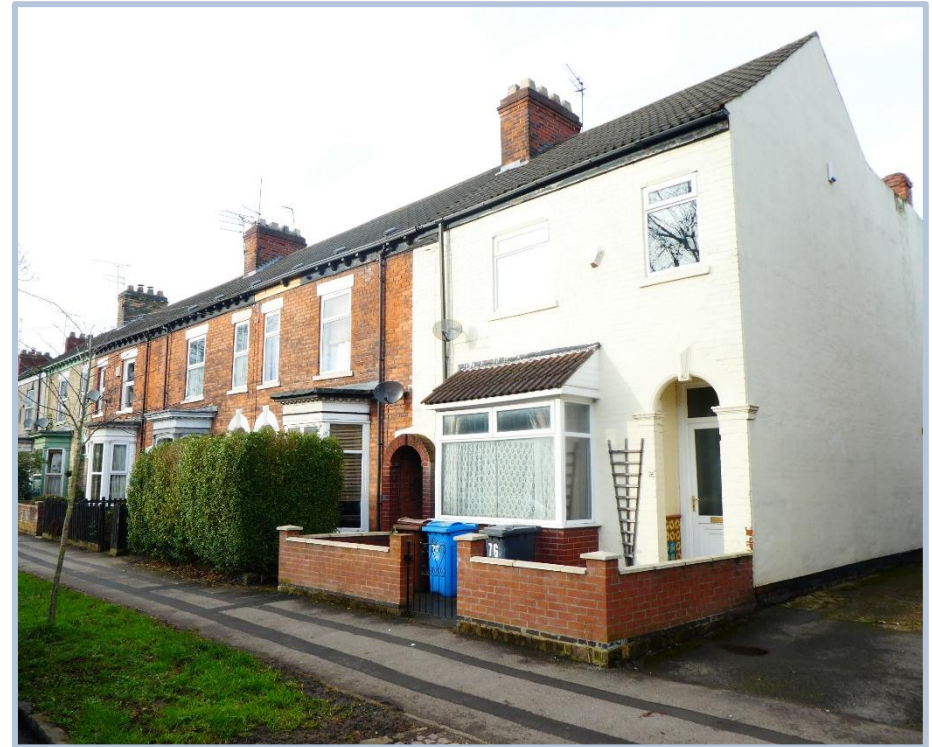
Figure 30. No.76 Ella Street, classified as a 'negative' building since the facade features including doors and windows do not match adjacent units and external rendering that deflect from the uniform character of the area.
