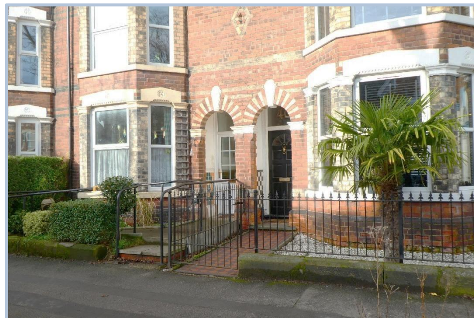
Figure 20. Brick facade and arch detailing.
