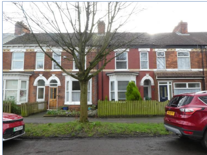
Terrace housing along Ella Street.
