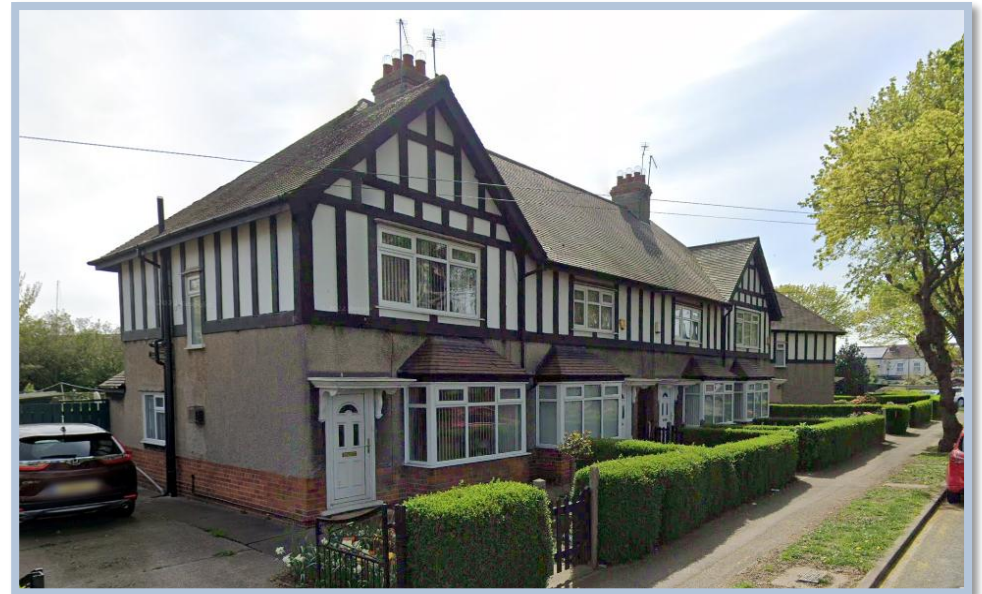
Figure 18. Short terraces along the junction of Seafield and Willows Avenue have similar features and appearance as demi-detached houses along Willows Avenue, but differ in length of elevation. Source: (Google Maps)
