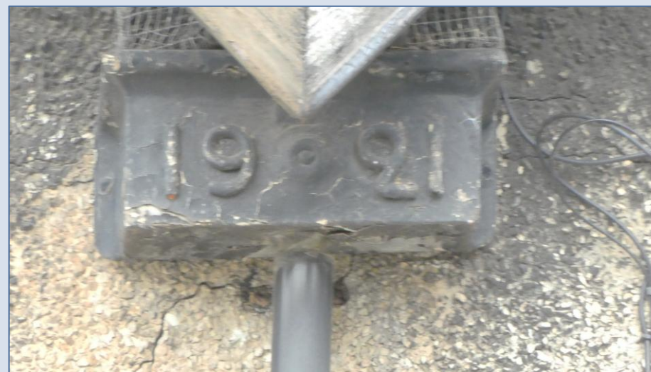
The 1921 original cast-iron rainwater gutter 'hopper' at 3-5 Seafield avenue is a distinctive feature, and only one of its kind within the area, and thus, desirable to be maintained.
