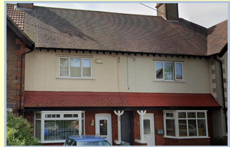
Figure 24. Variety of roof materials within the Conservation Area. Source: (Google Maps, 2022)
