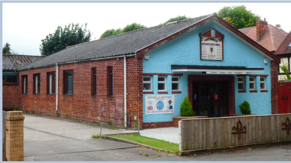
Figure 19. Portobello Methodist Scout Group HQ. Source: (Walker, 2024)
