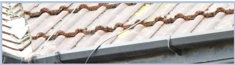
Figure 13. Zoomed in picture of double roman pantiles. Source: (Walker, 2024)
