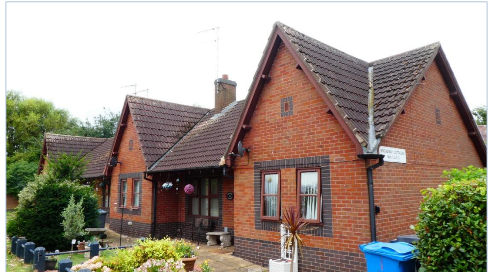
Figure 22. Rear elevation of Broadway Cottages. Source: (Walker, 2024).
