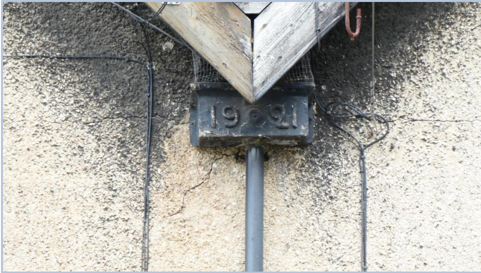
Figure 28. Original cast-iron rainwater goods at 3-5 Seafeld Avenue.
