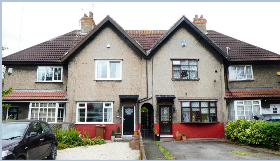
Figure 10. 1-7 Seafield Avenue, style 6. Source: (Walker, 2024).
