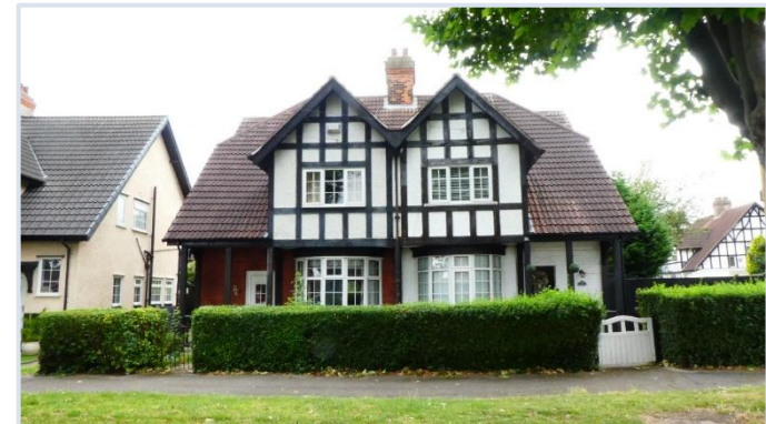
Figure 4. House no.s 18-20 The Broadway, designed in Style 1 of the BOCM layout. Source: (Walker, 2024)
