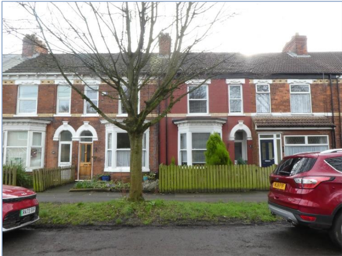
Terrace housing along Ella Street.
