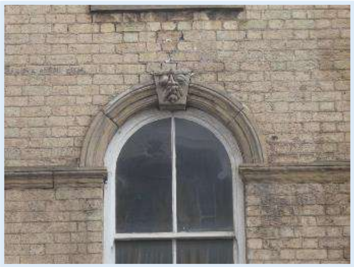
Figure 73 Decorative Lintels, on Paragon Street
