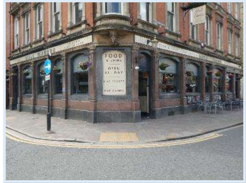
Figure 57 – Victorian frontage at Hull Cheese, Chapel Street & Paragon Street
