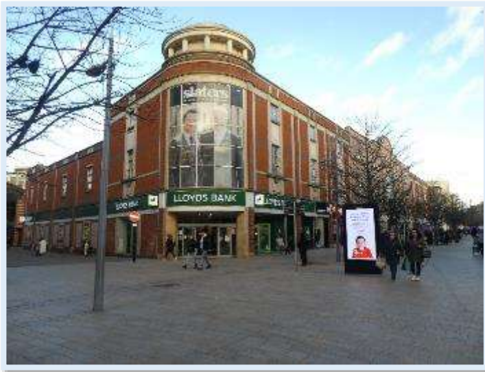
Figure 88 1990s Grand Buildings, Jameson Street
