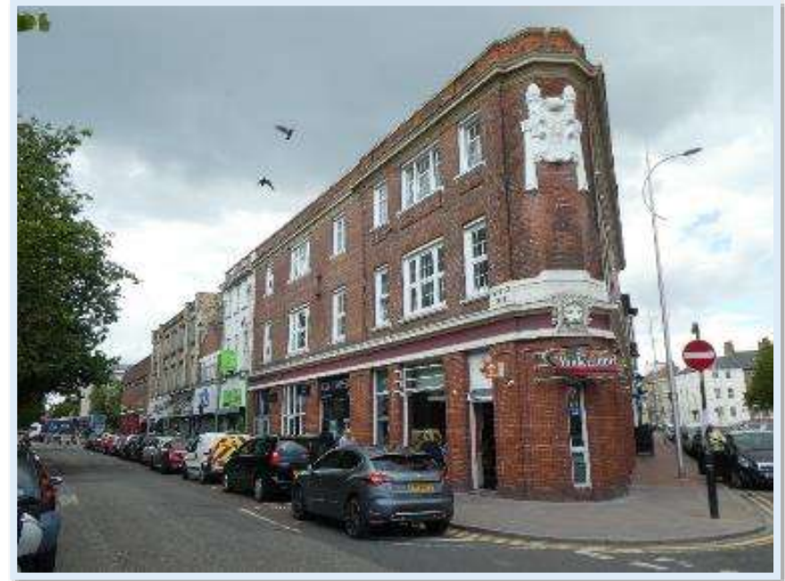
Figure 81 Positive Buildings along Prospect Street
