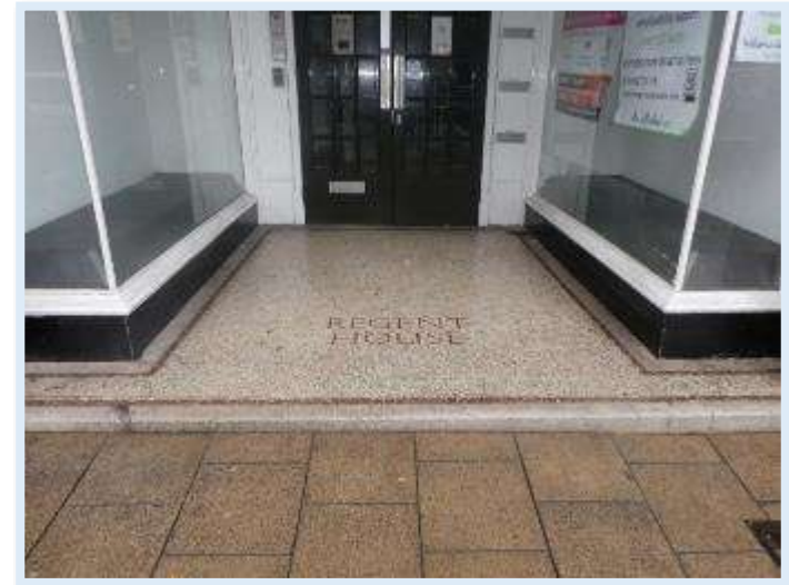
Figure 75 Entrance Lobbies, such as at Regent House.
