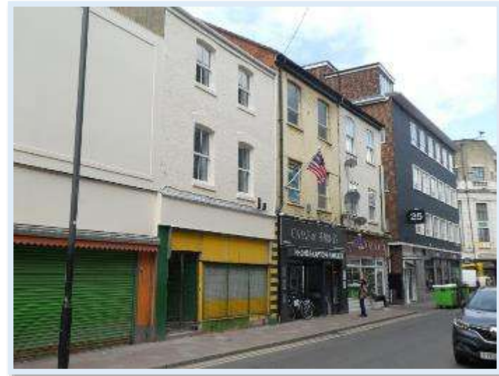
Figure 65 Appropriate and in-appropriate uPVC replacements windows on South Street
