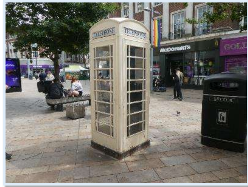
Figure 105 K6 Telephone Box, Jameson Street
