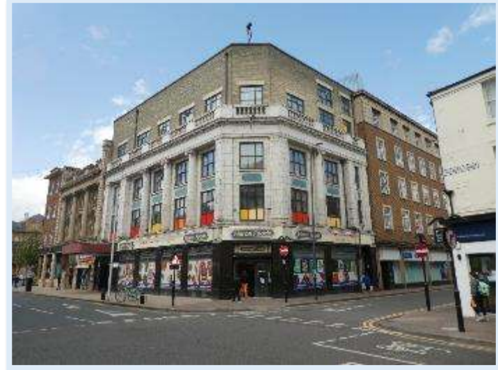
Figure 79 Former Jacksons Store, Paragon Street
