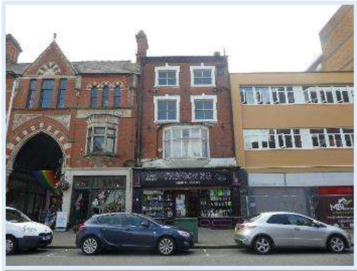
Figure 63 Historic Sash windows 55 Paragon Street
