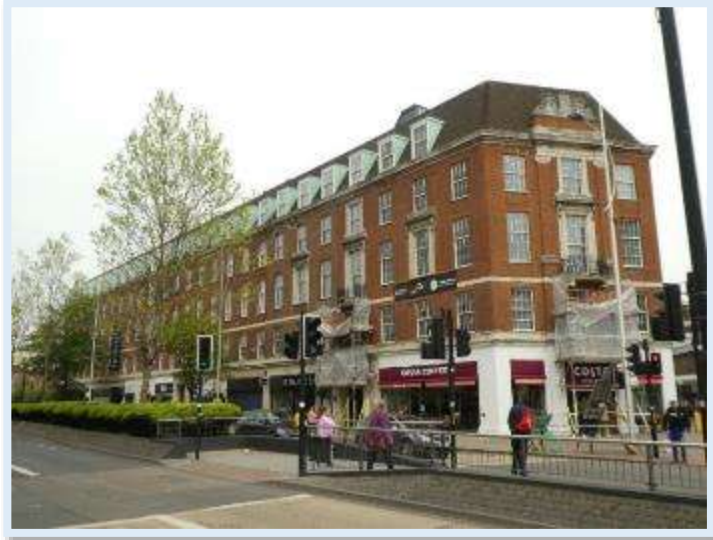
Figure 25 Local Listed Brook Chambers, Ferensway Chambers & Debenhams, Ferensway
