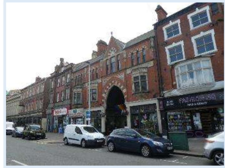
Figure 85 Key and Positive Buildings along Paragon Street
