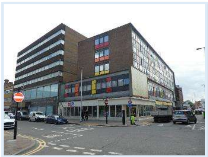
Figure 89 Former Portland Hotel and Tivoli House, Carr Lane
