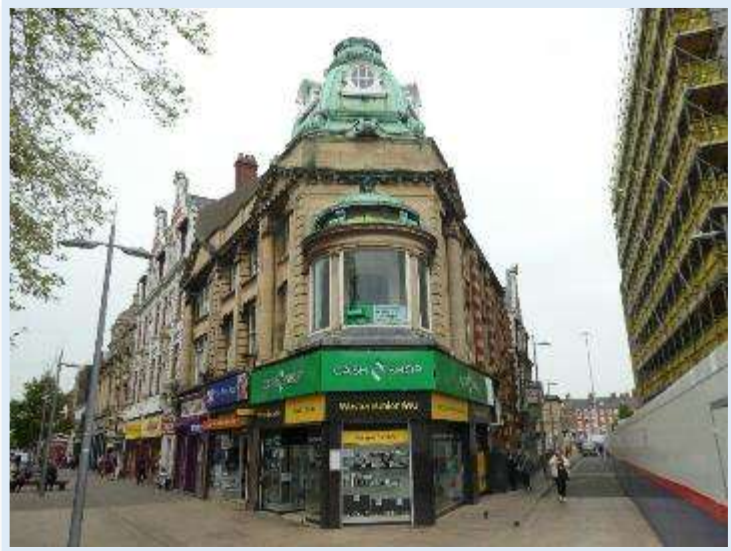
Figure 22 Grade II 46, 48 & 50 King Edward Street
