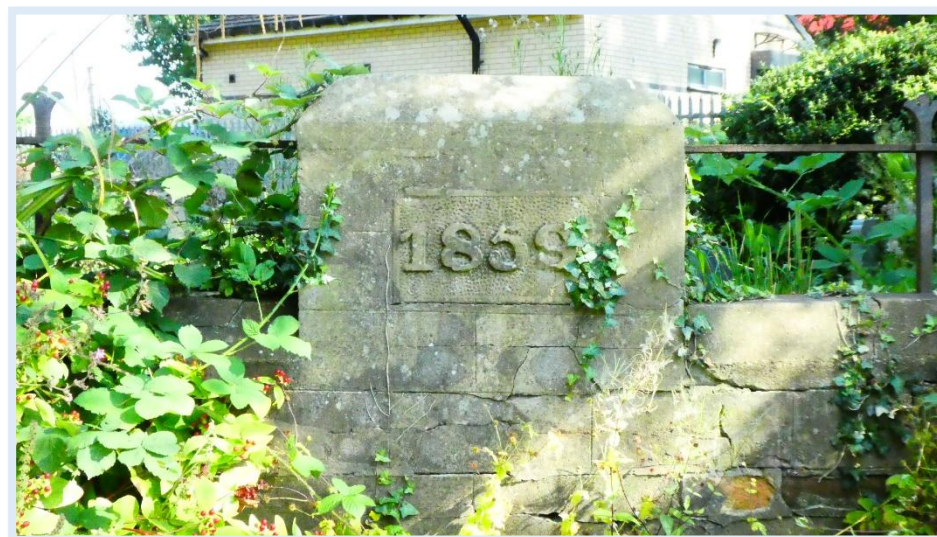
Figure 25 - Date stone located within the Grade II listed boundary wall to the Church Yard.
