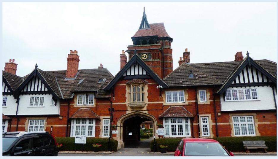
Figure 100 - The principal facade of Northumberland Court (Grade II).
