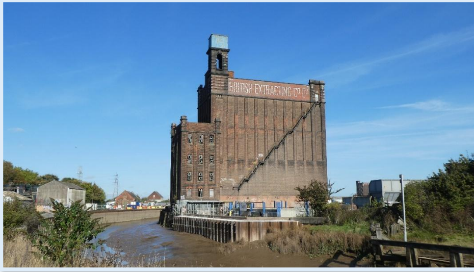
Figure 53 - Former B.E.C. Silo & attached Receiving House, Foster Street (Grade II).
