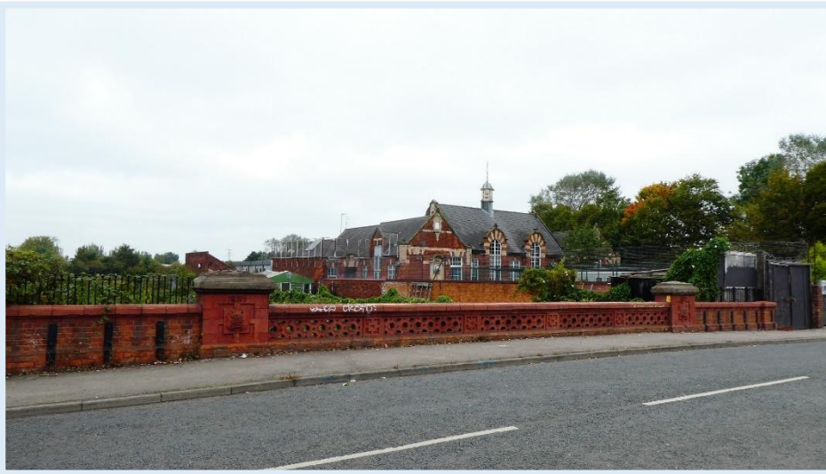
Figure 28 - Fountain Road Bridge (Locally Listed)
