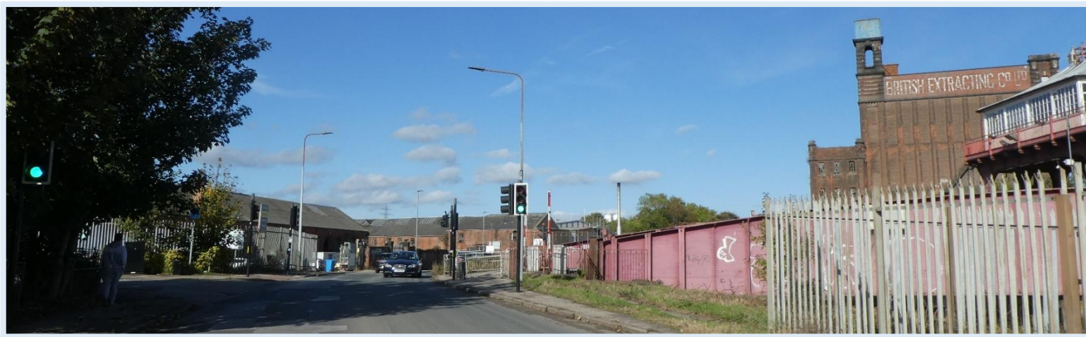
Figure 48 - The remaining Victorian & Edward elements of Sculcoates.
