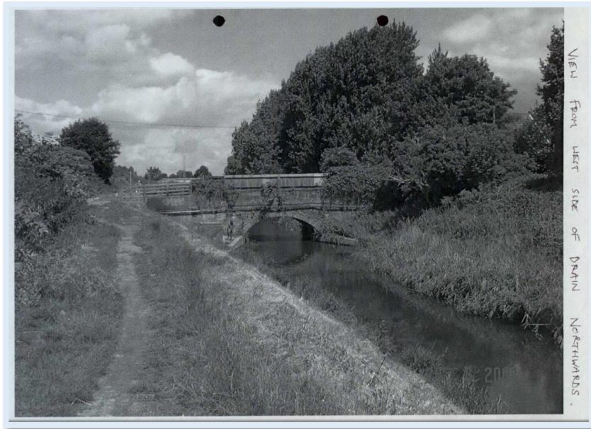
Figure 17 - Character of the drain before the implementation of application 04/00941/FULL.
