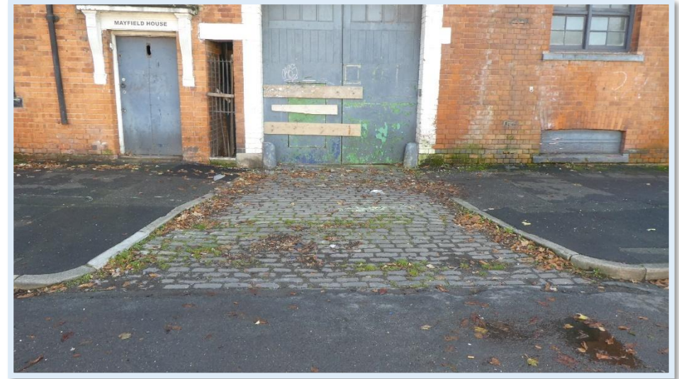
Figure 72 - Setts at the former Paint Warehouse, Sculcoates Lane.
