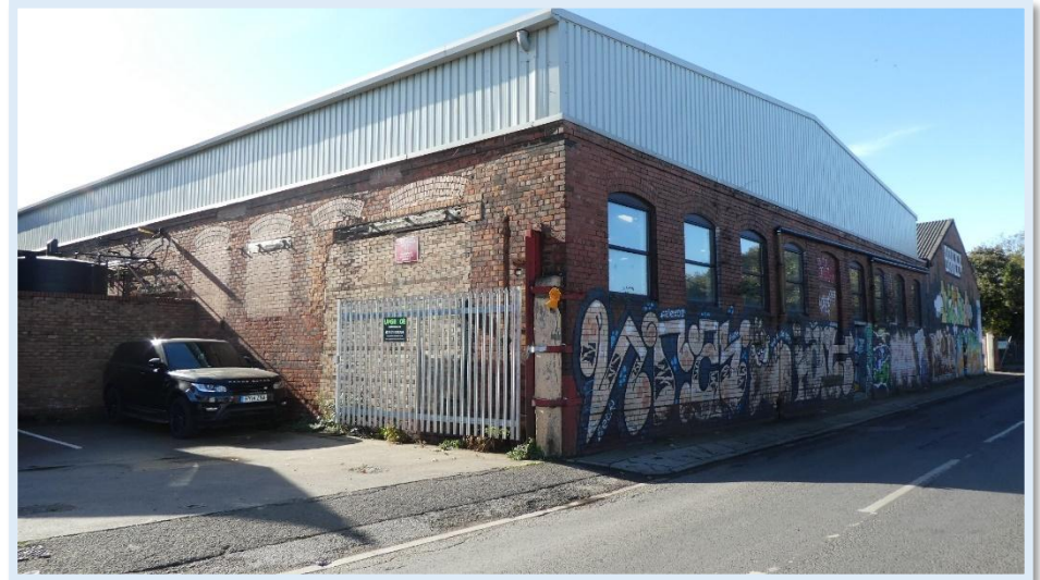
Figure 56 - Retained facade of 'Tan Pits' on Air Street.
