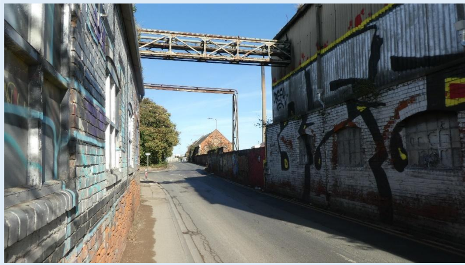
Figure 68 - Enclosure formed by historic buildings facades along Wincolmllee.
