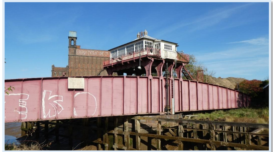
Figure 52 - Wilmington Railway Swing Bridge (Grade II).
