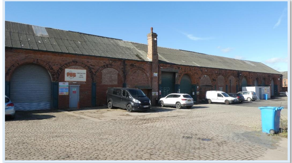
Figure 51 - Former Sculcoates Station Goods Shed, Wincolmllee (Grade II).
