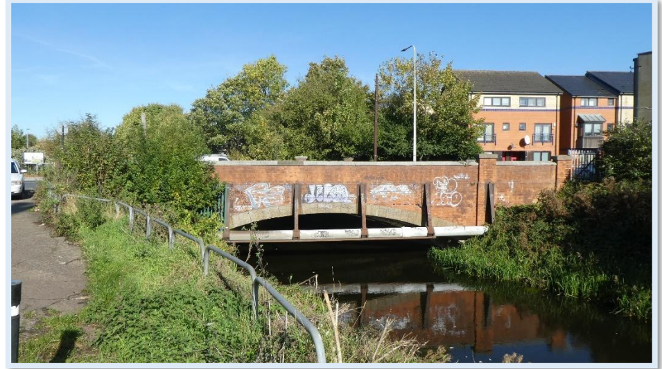
Figure 34 - Sculcoates Lane Bridge
