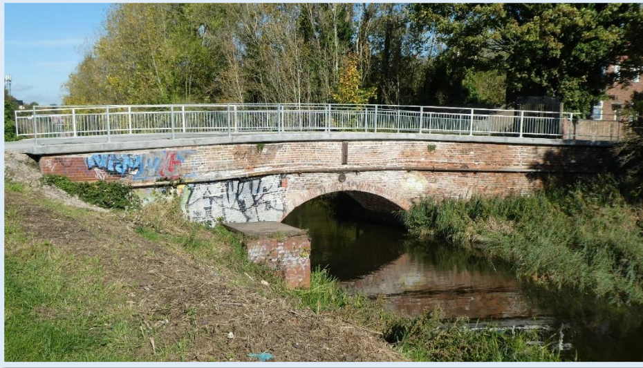
Figure 27 - Stepney Lane Bridge (Locally Listed)
