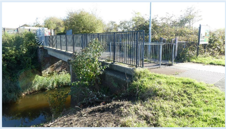
Figure 33 - The current bridge deck, built on 19th century railway bridge footings.
