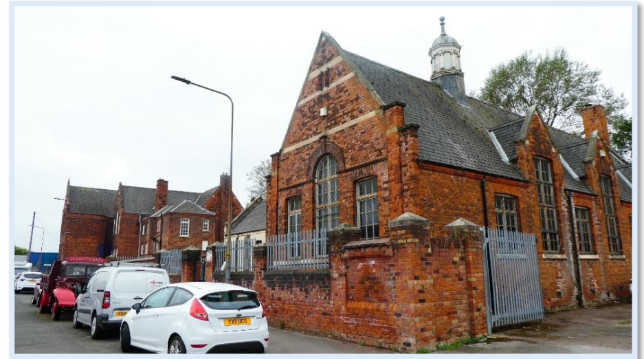
Figure 106 - View without visible modern development.
