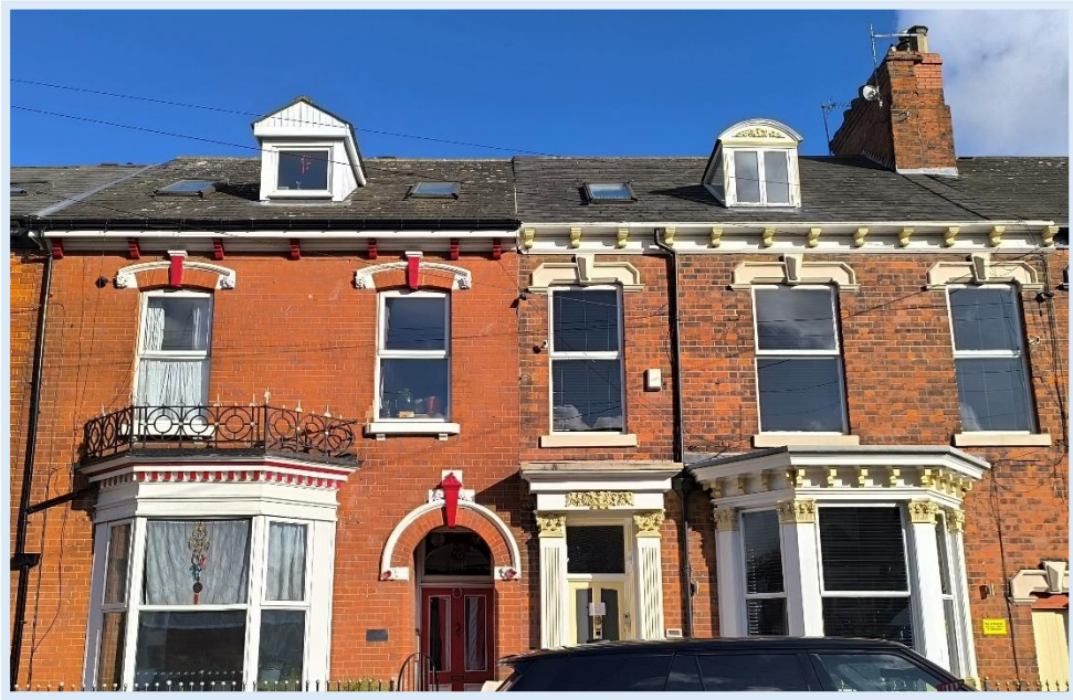
Figure 18. Decorative eave details. Source: Author.
