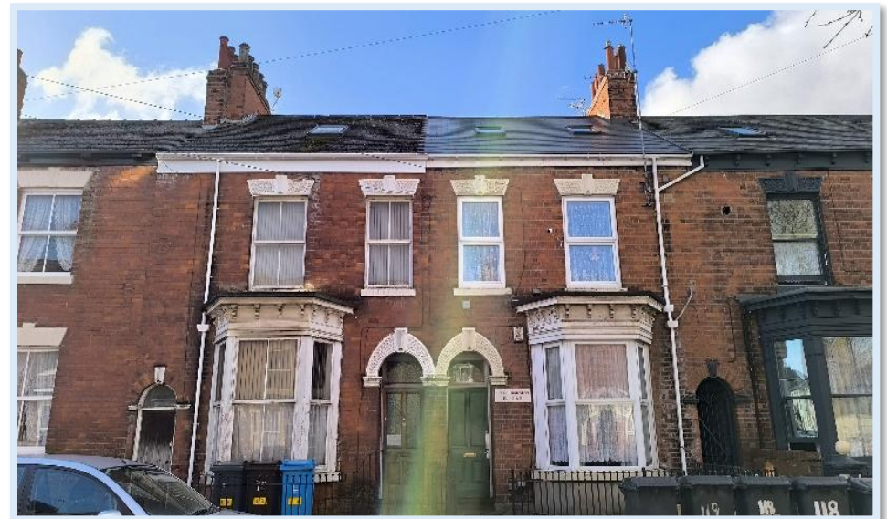
Figure 25. Proliferation of rooflights observed in the area.
