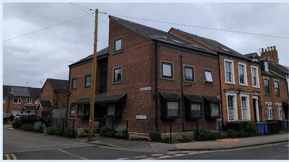
Figure 24. Negative window type - not in scale, type and proportion in comparison to other 'positive' windows of the conservation area.
