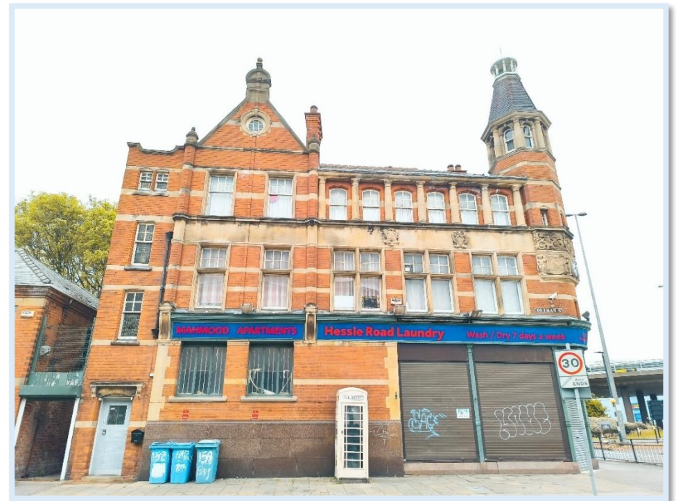
Figure 30. Focal entrance buildings.
