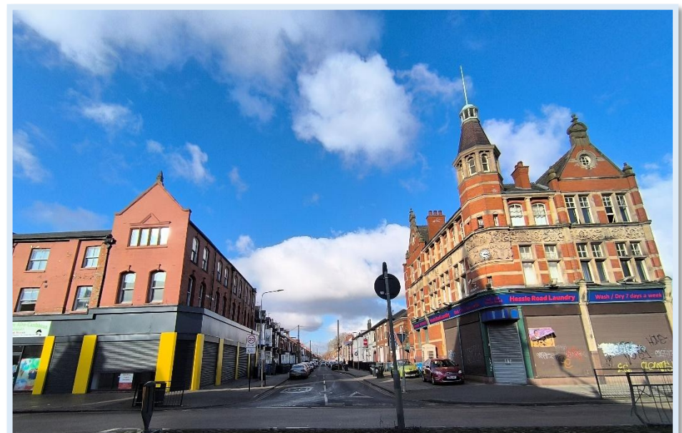
Figure 31 - . Negative shopfronts on listed and focal buildings.
