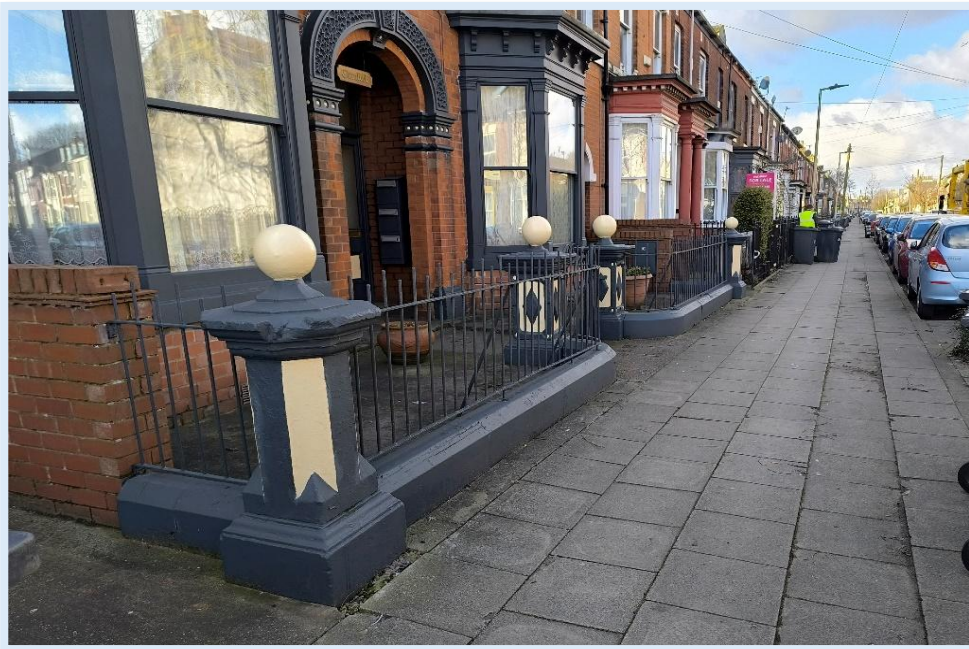
Figure 17. Hexagonal stepped pier with ball finial at 121 Coltman Street.
