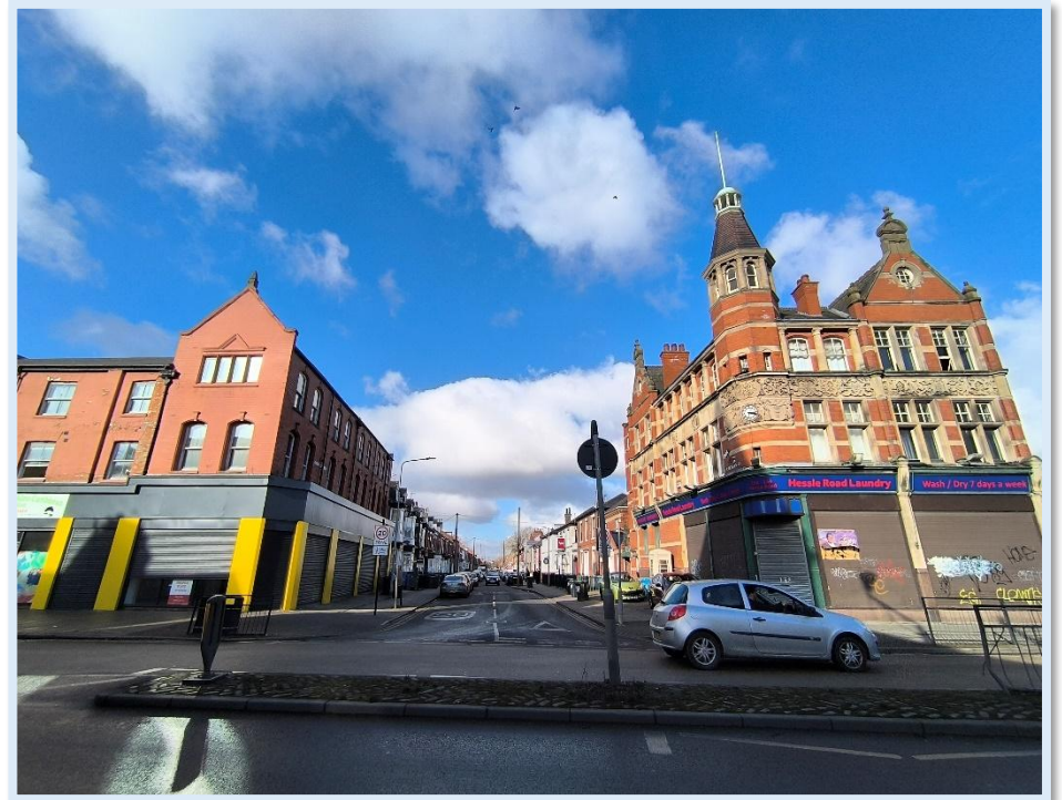
Figure 28. Negative alterations to focal buildings.
