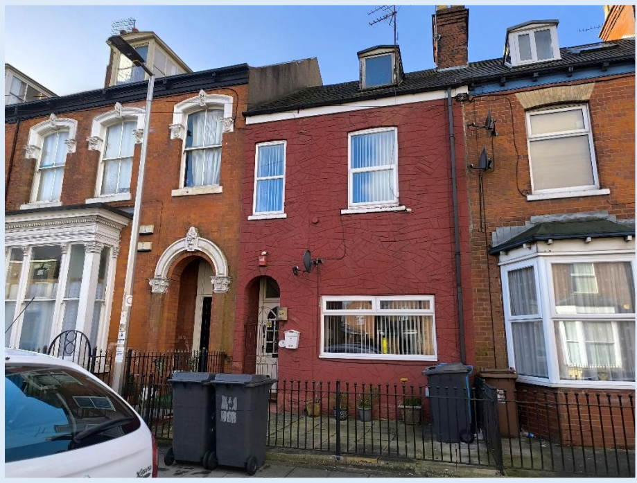
Figure 26. Negative element - External rendering at 146 Coltman Street.
