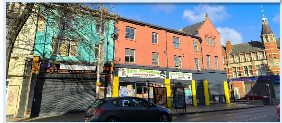
Figure 27. Negative shopfronts on focal buildings.
