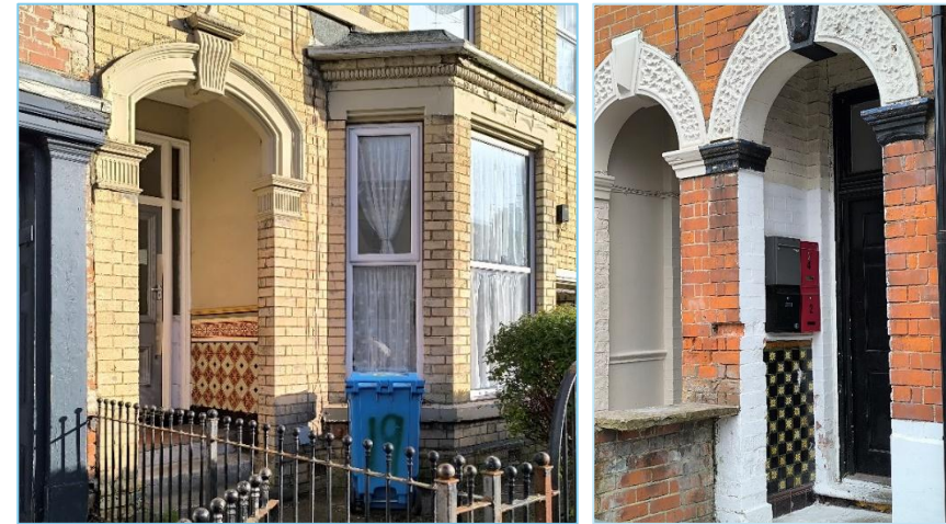
Figure 21. Glazed wall tiles inset within entrance porch.
