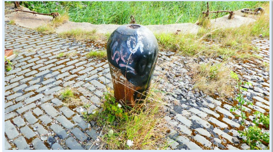
Figure 33 - Mooring Post and Dock Side 'Sett' surfacing.
