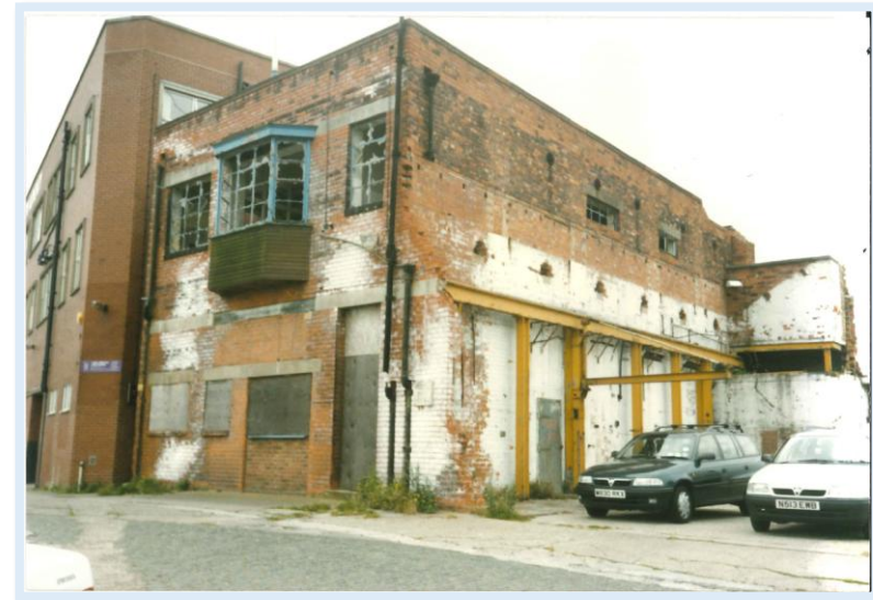
Figure 47 Former 'Gas Engineers' Office shown in 1997. Approved for demolition in 2012.
