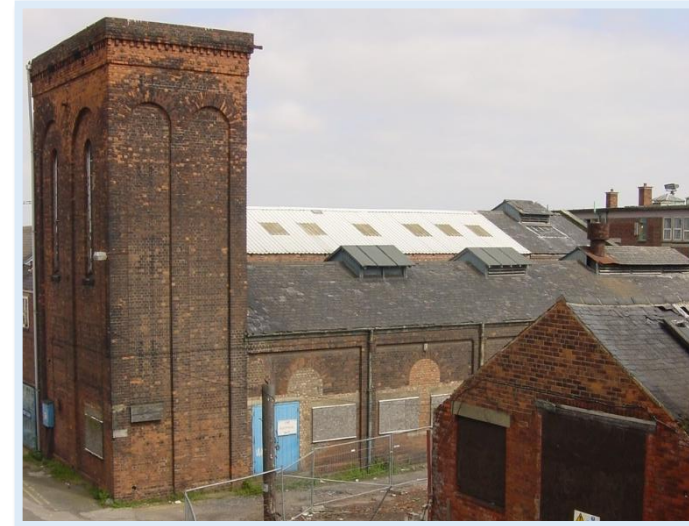
Figure 22- Hydraulic Tower and Pump House in 2011.
