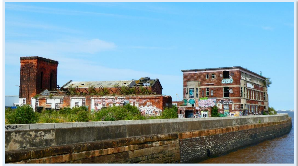
Figure 53 - Grade II listed Hydraulic Tower & Pump House, and Insurance Building.
