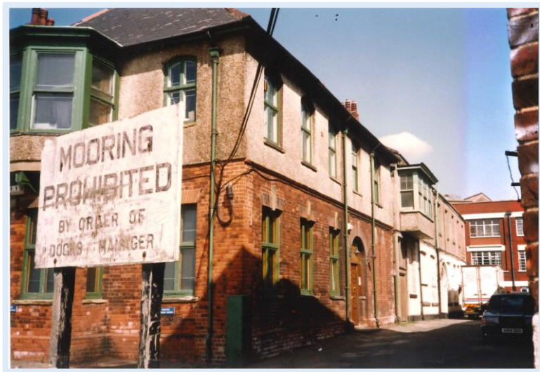
Figure 49 Glimpsed view towards the J. Marr Building, with the Albert Club in the foreground. Photographed in 1992.
