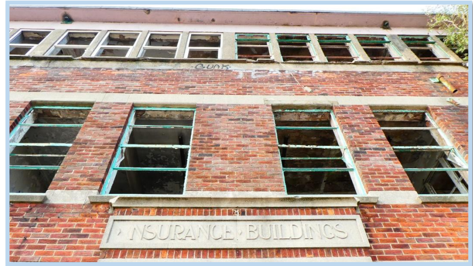
Figure 38 - Stone detailing and remaining window details at the Insurance Building.
