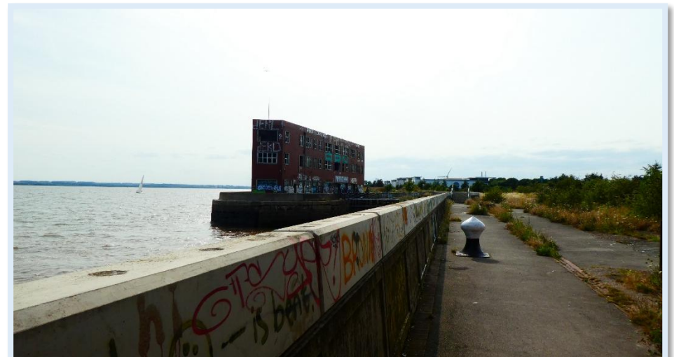
Figure 37 - Enclose of the dock by the flood wall & impact upon the function of the mooring posts.
