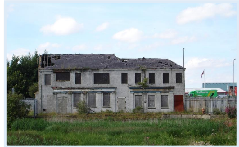
Figure 46 Bank Building 2007. Approved for demolition in 2012.
