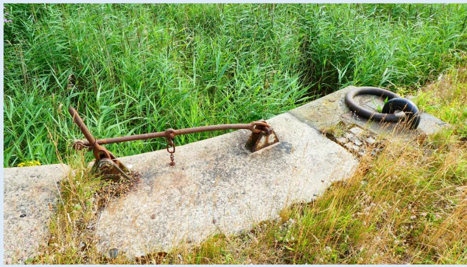
Figure 17 - Visible section of the remaining dock wall and mooring ring.
