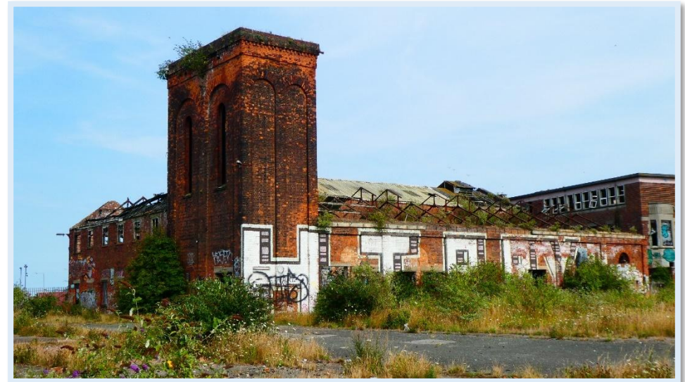
Figure 23 - The Hydraulic Tower and Pump House in 2024.
