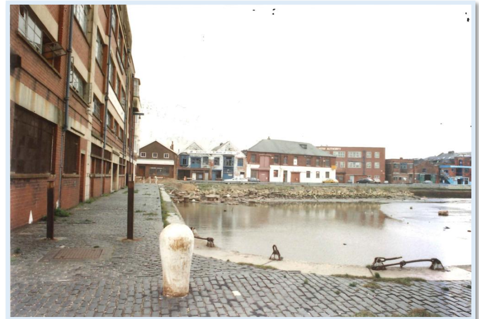
Figure 10 View of Lord Line Building, Dock and 'Triangle Plot' in 1991.
