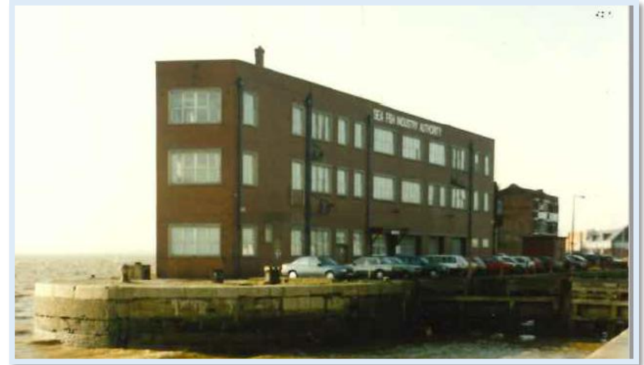
Figure 30 Steam Fishing Building in 1998.
