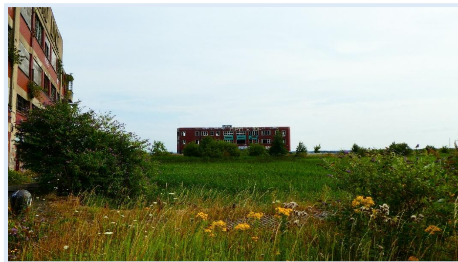
Figure 3 - View towards the Fisheries Building, showing the in-filled dock.
