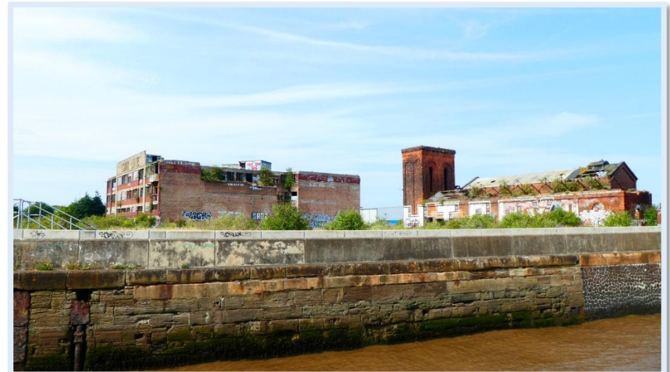
Figure 21 - St Andrew Dock River Wall in 2024.
