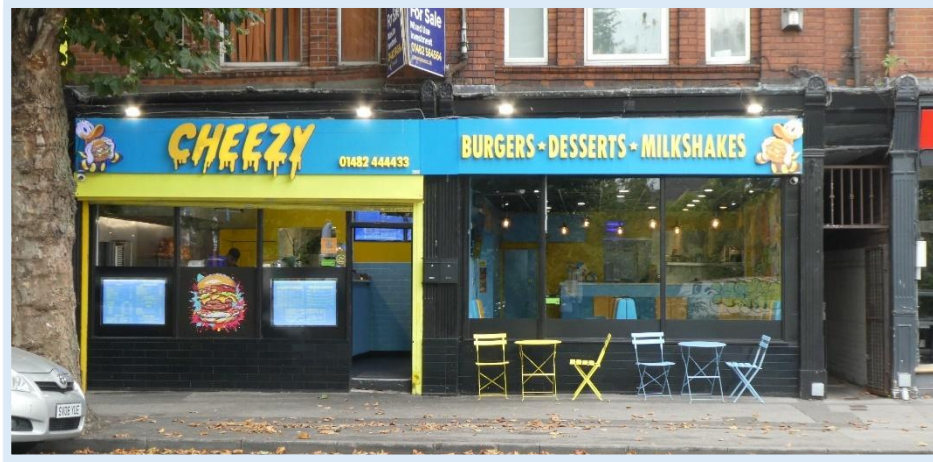
111 - Unauthorised alterations to Nos.21-23.
