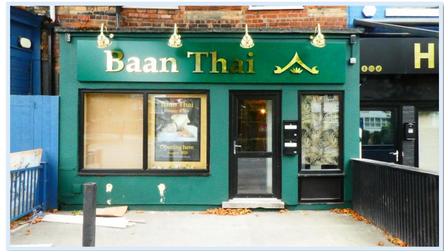
68 - None traditional shop front at No.66.
