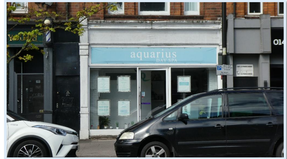
54 - Nos.27-29 Retained historic shop surrounds but modern shop windows.
