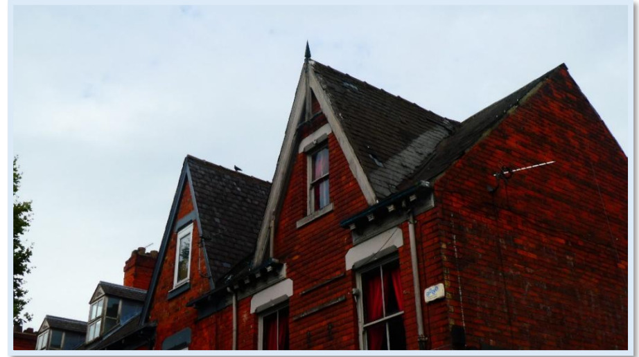
21 - Pitched gables and barge boards at Nos.12a-28.
