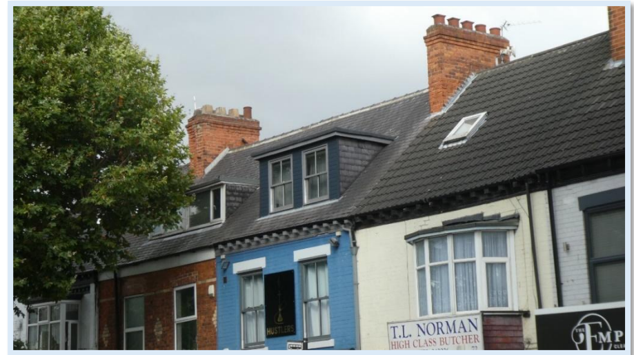
27 - Historic and new roofing materials, chimneys, and none-historic dormers.
