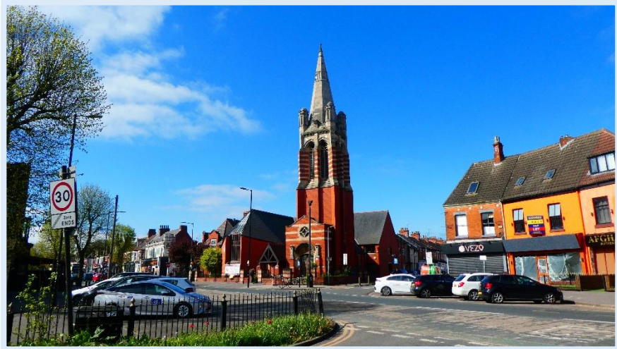
93 - Primitive Methodist Church from Park Grove.
