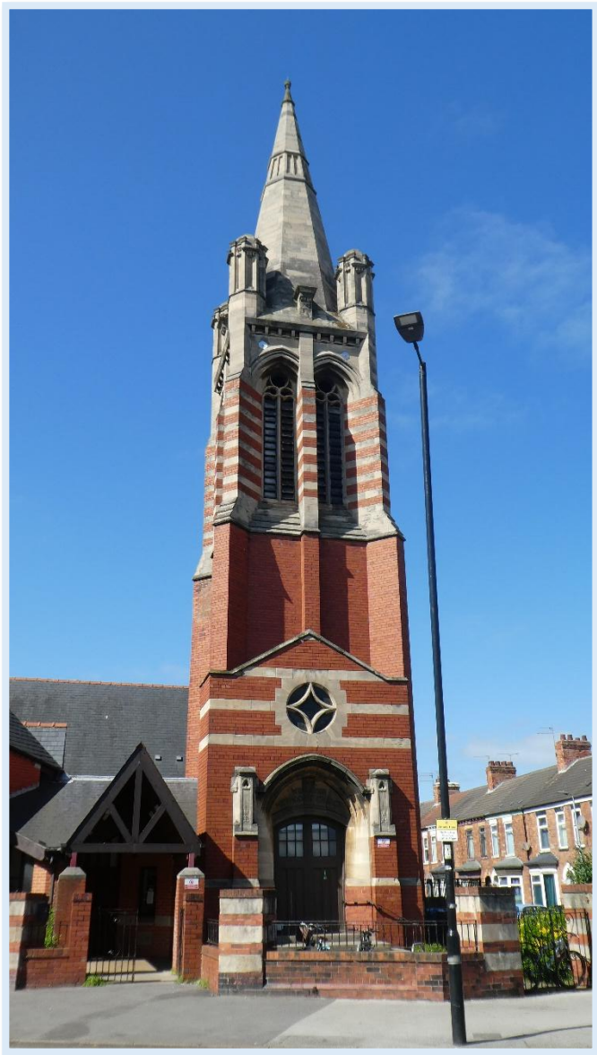
100 - Grade II - Primitive Methodist Chapel Tower.
