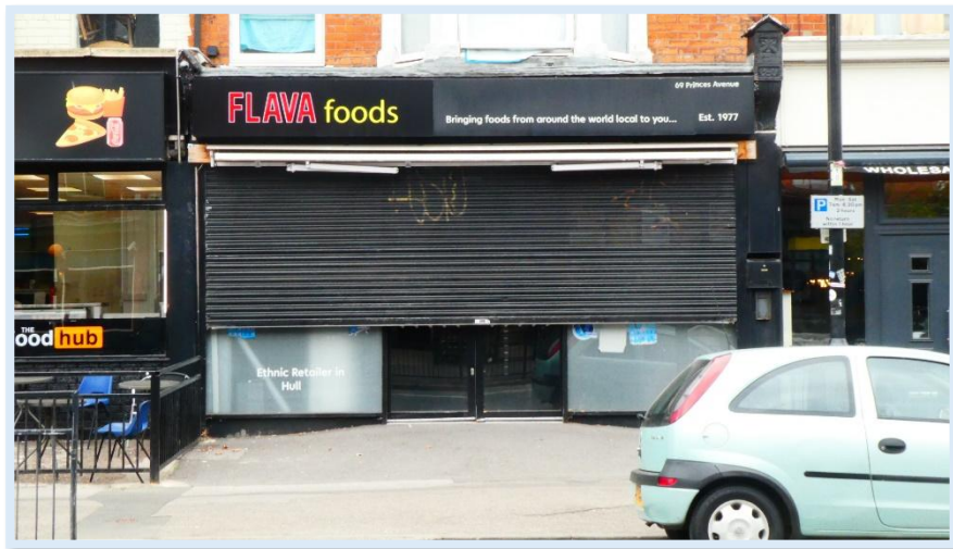
75 - Unauthorised Roller Shutter at No.69.
