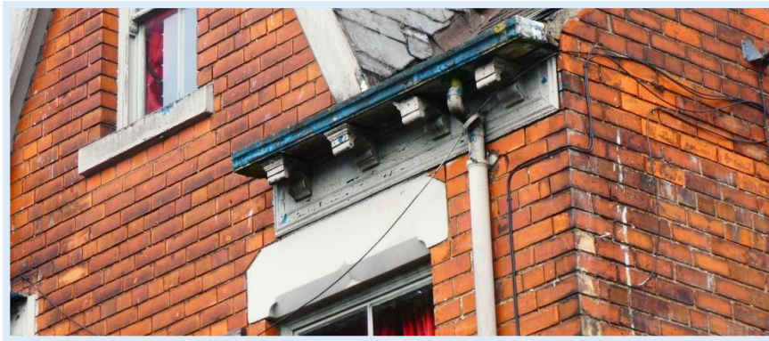
29 - Typically form of rainwater goods at No.12a.
