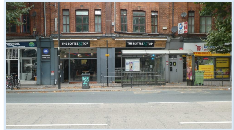
61 - Negative elements adverts and design at Nos.13-15 but retained historic pilasters.
