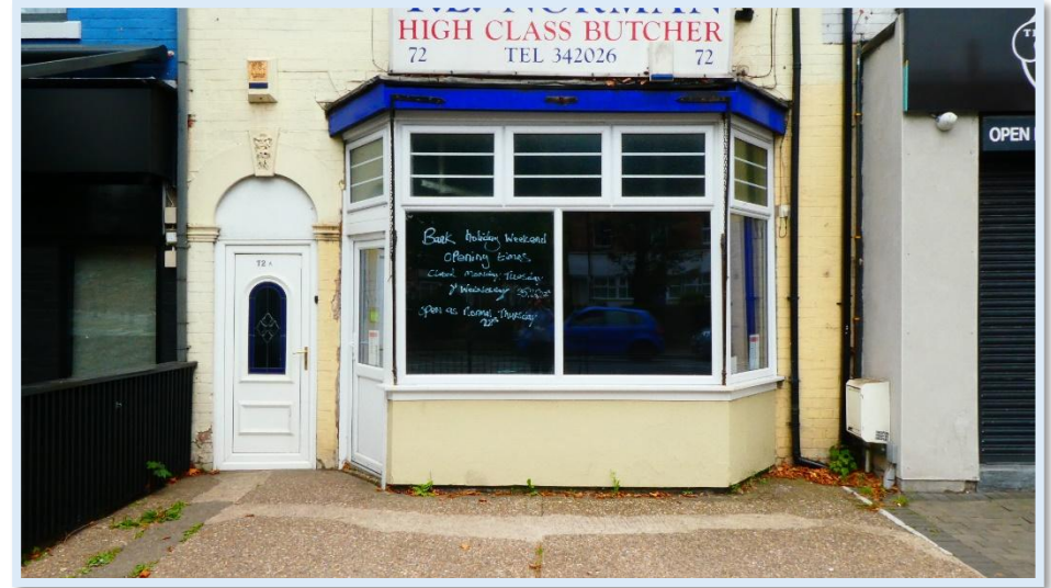
73 - No.72 retains its historic form but now feature uPVC glazing.
