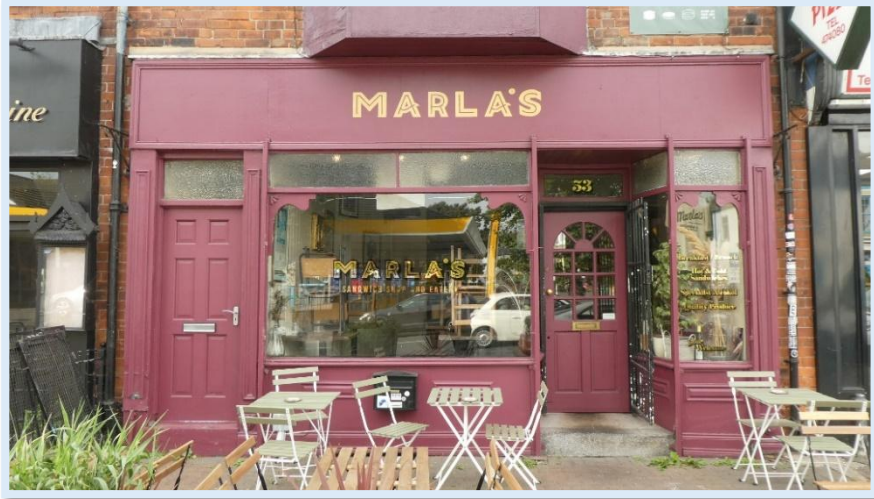
51 - No.53 - Positive quality shop front restoration.
