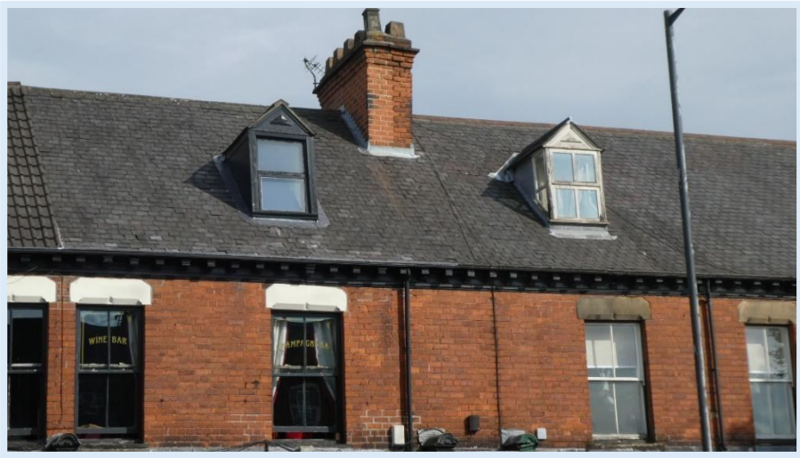
25 - Slate tiles, timber windows, traditional dormers and chimney at Nos.12-28.
