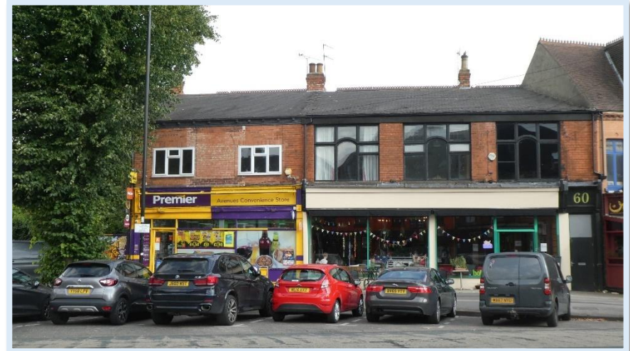
117 - Approved shop front alterations at Nos.60 & 62, and advertisement clutter.
