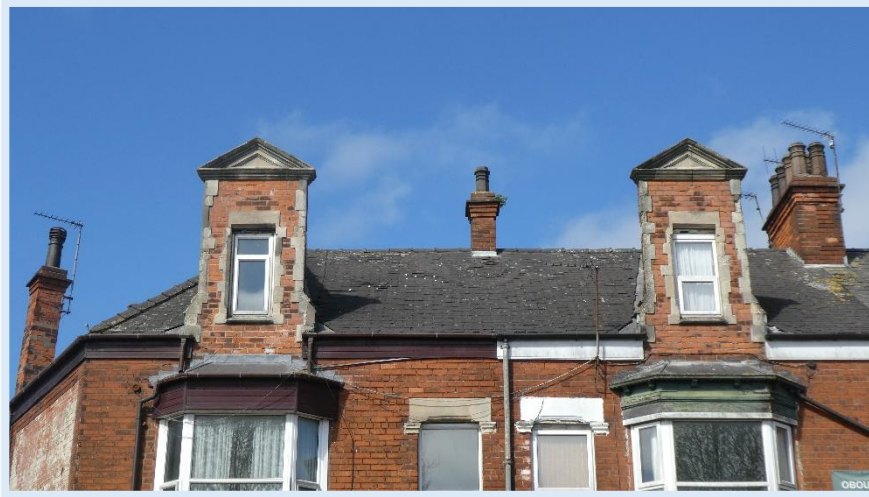
20 - Roof slates and dormers at Nos.51 and 53.
