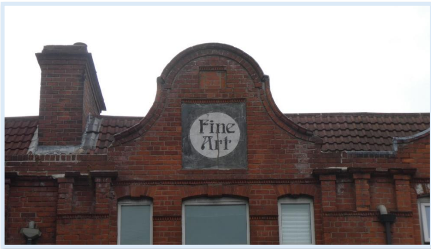
83 - First floor advertising at Nos.7-43.
