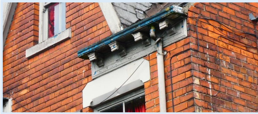
29 - Typically form of rainwater goods at No.12a.
