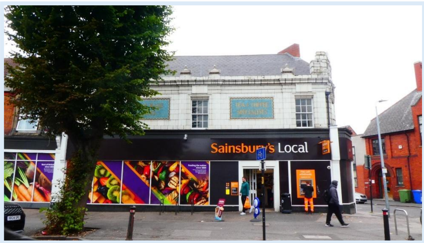
124 - Negative quality of in-active shop fronts at no.83-85.
