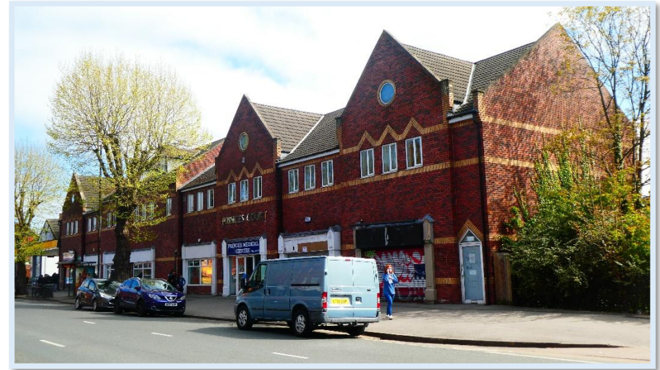
104 - Princes Court neutrally contributes towards special interest but includes positive architectural elements.
