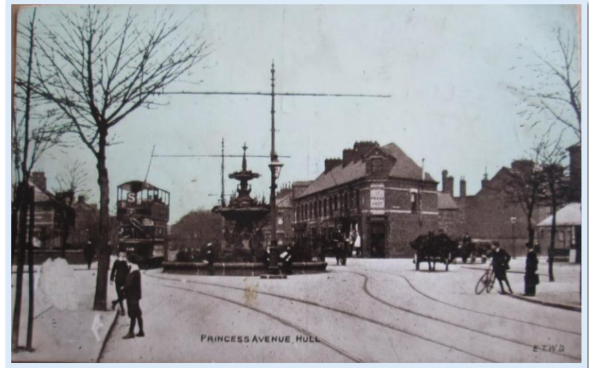
Figure 5 - View towards No.70 Princes Avenue.
