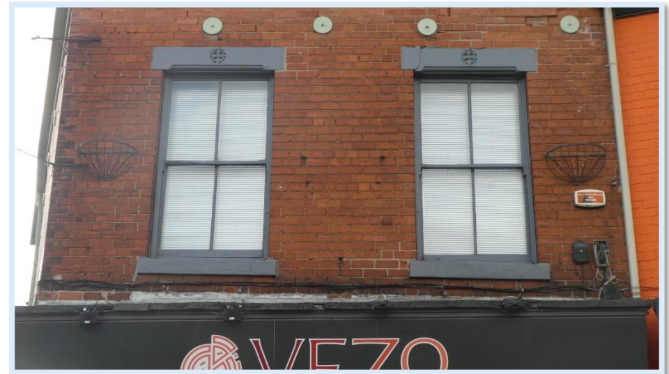
28 - Good quality timber 2/2 windows at No. 93.
