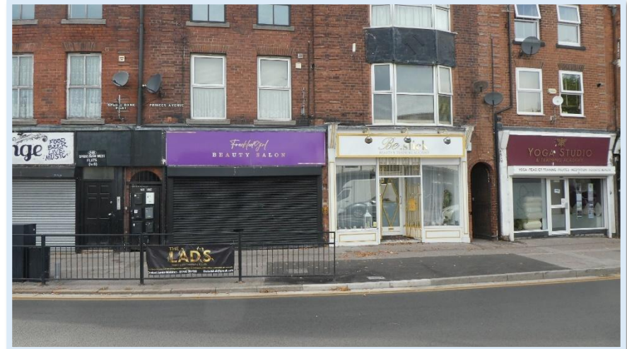
116 - Introduction of Roller Shut hides the architectural value of No.1 Princes Avenue.
