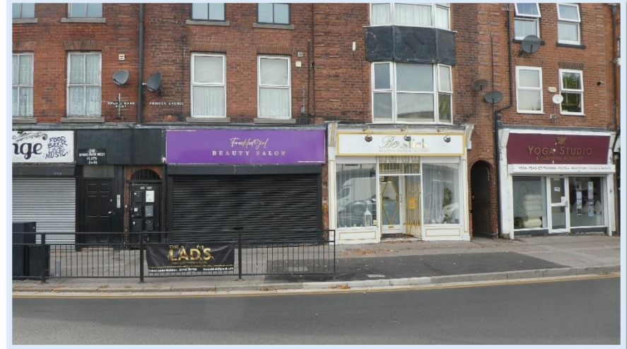
116 - Introduction of Roller Shut hides the architectural value of No.1 Princes Avenue.
