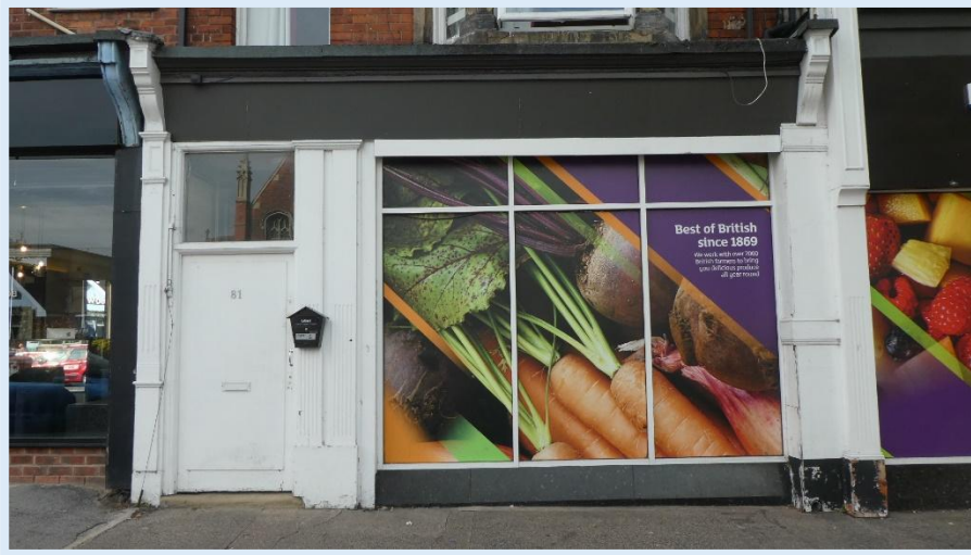
52 - Historic element of No.81 are retained.
