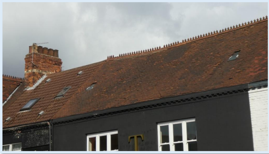
24 - Clay tiles with ridge tiles and contrasting modern materials.
