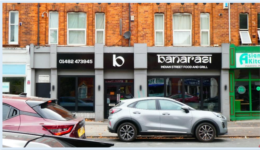
66 - Out of scale pilasters and capitals at Nos.31-33.
