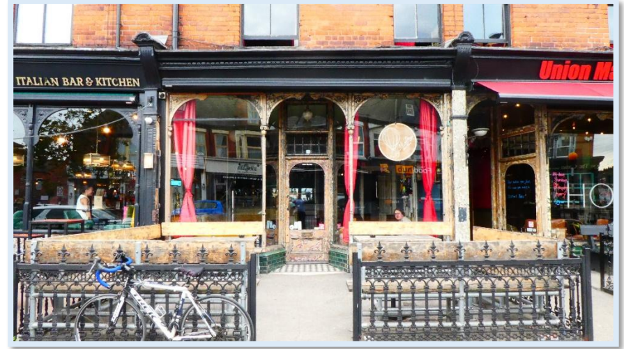
44 - No.24, partially obscured by fixed external seating, with unauthorised awning.
