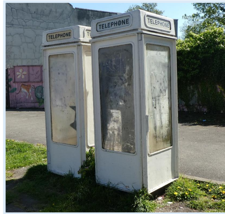
Figure 98 - Pair of Grade II K8 Telephone Boxes. Condition is a concern at time of survey.
