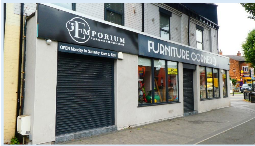
62 - In-active shop frontage at No.70.
