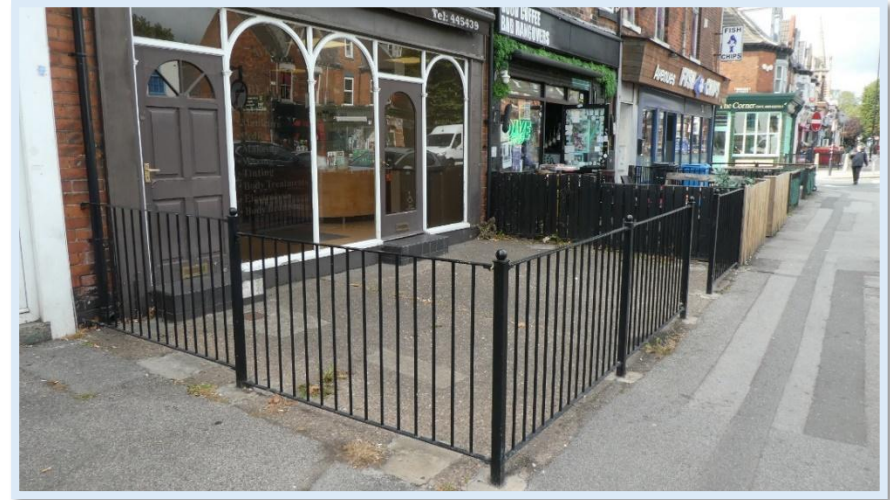
80 - No. 57 - The lightweight railings maintain the view of the shop front and is free of 'clutter'. Timber boundaries contribute negatively.
