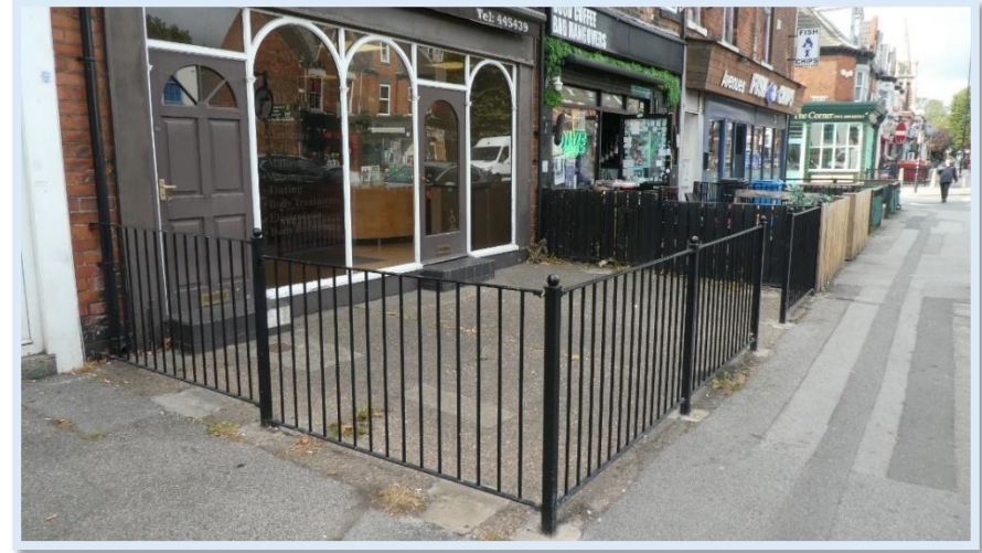
80 - No. 57 - The lightweight railings maintain the view of the shop front and is free of 'clutter'. Timber boundaries contribute negatively.
