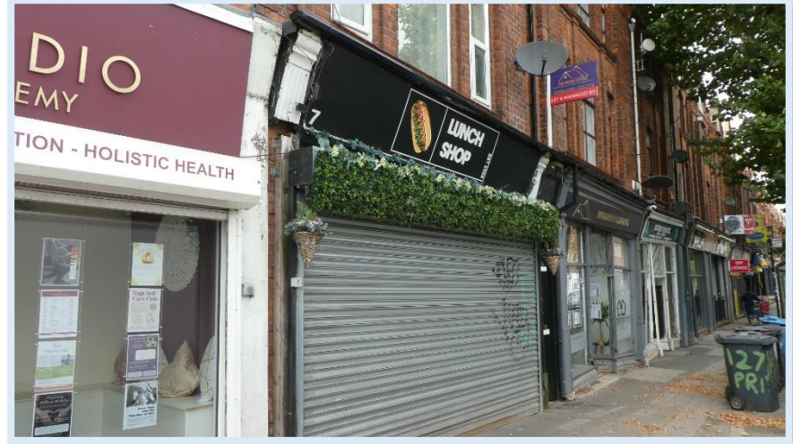
39 - Nos.7-11 - Historic shop front, harmed by the introduction of a roller shutter.
