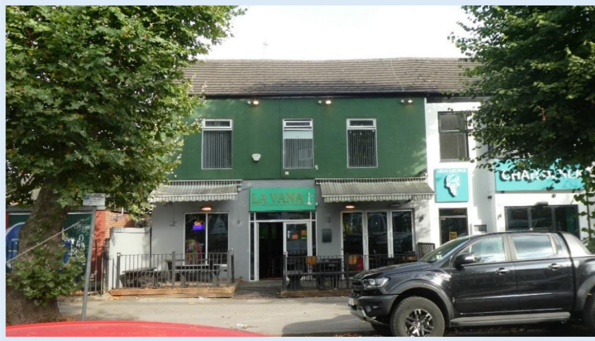
119 - Approved shop fronts at No.82 and 84, and unauthorised works at 84.
