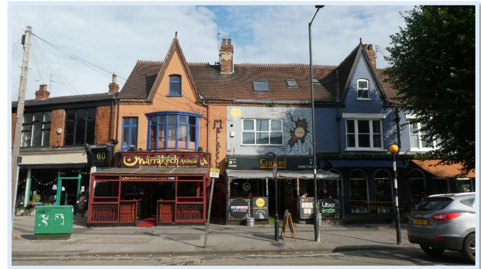
Figure 113 - Nos. 58 & 56 Princes Avenue in August 2025 with part approved development and unauthorised works. Also with negative first floor advertisements.
