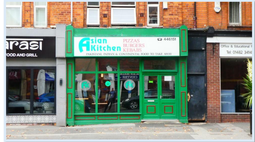
53 - Good quality shop front restoration but does not re-instate group value.
