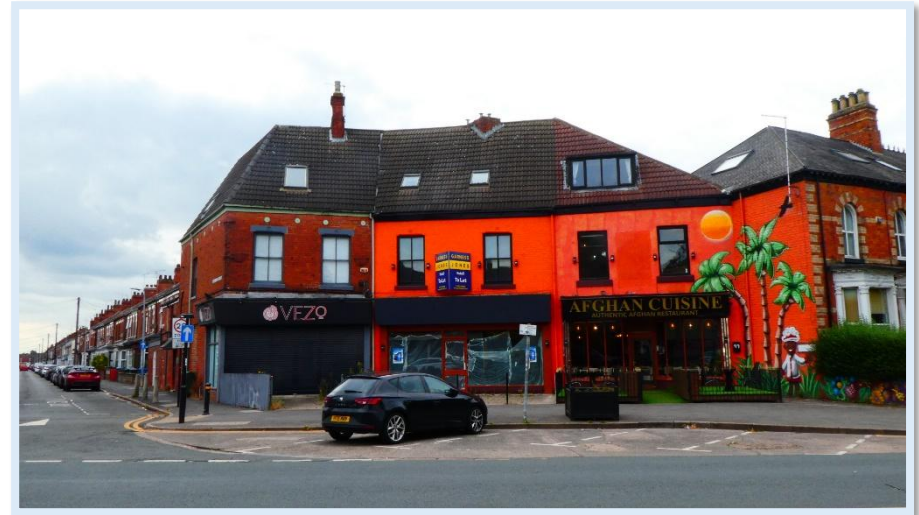
30 - Loss of uniform design and material use at Nos.93-97.
