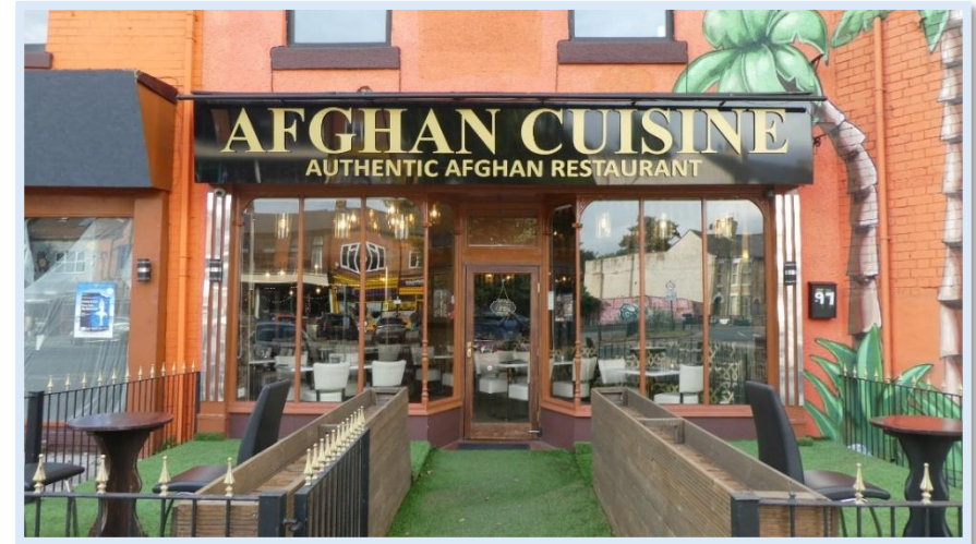
48 No. 97 after alteration in August 2025.
