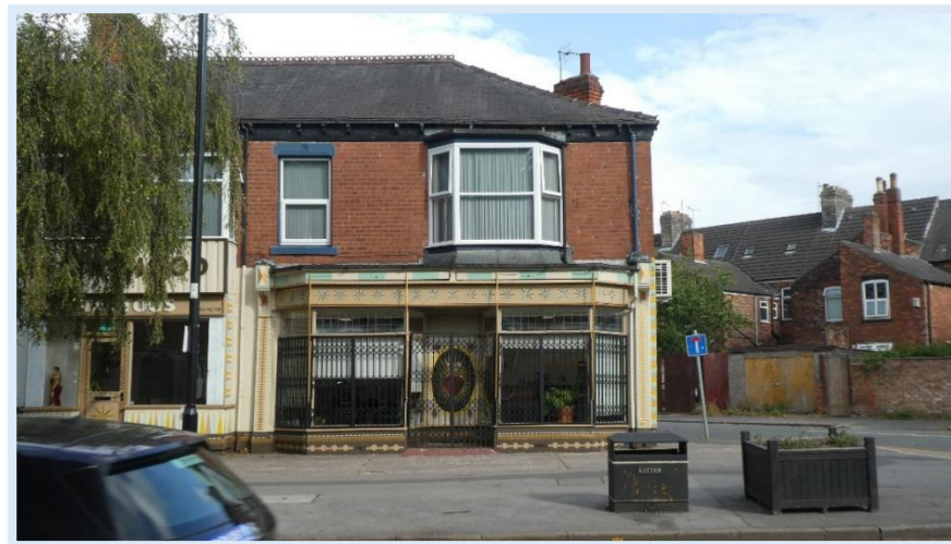
101 - No.80 - One of the best surviving shop fronts within the Conservation Area.
