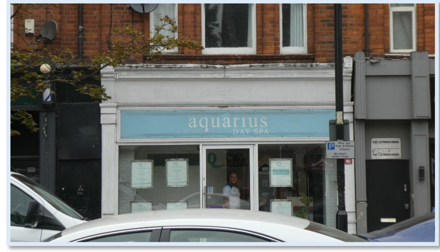
54 - Nos.27-29 Retained historic shop surrounds but modern shop windows.
