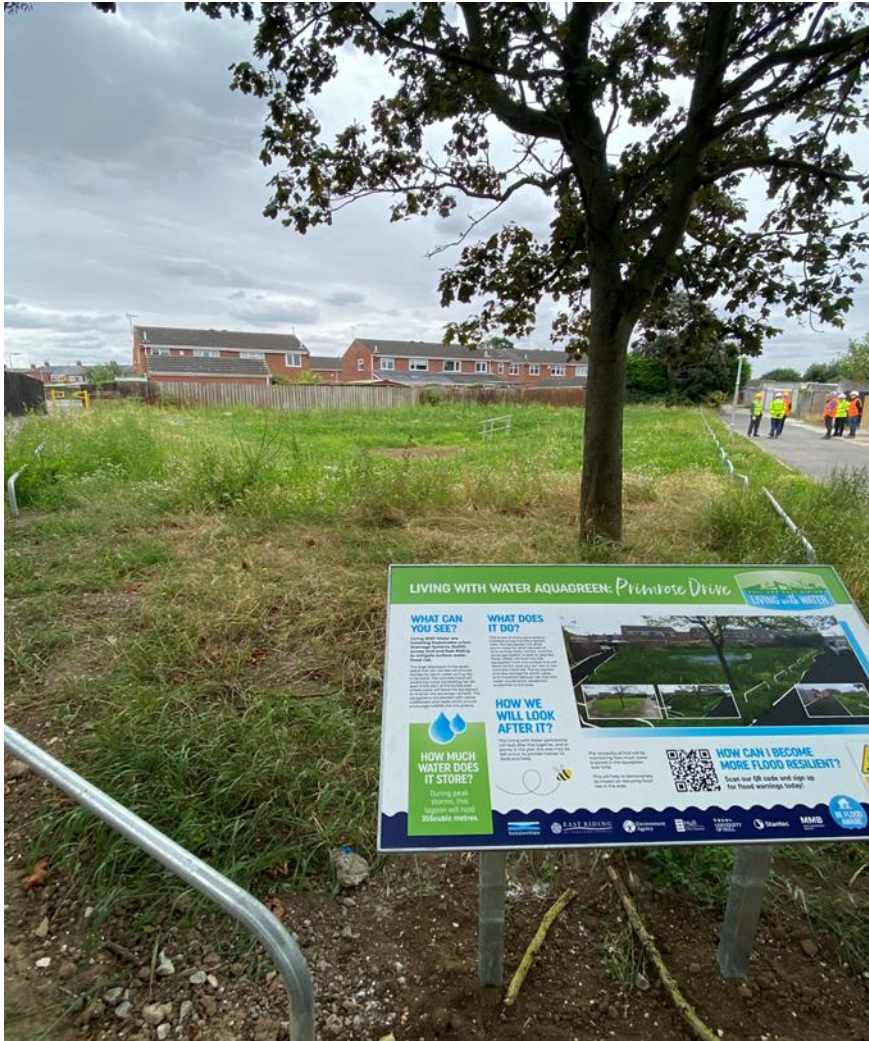
Example of BNG incorporated into a SuDs retrofit at Primrose Drive, Derringham Hull.
