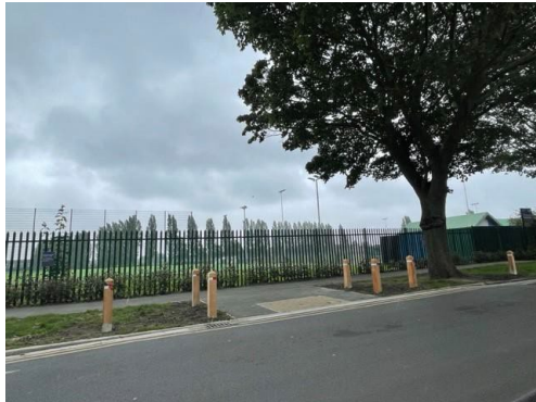
Bollards on Inglemire lane
