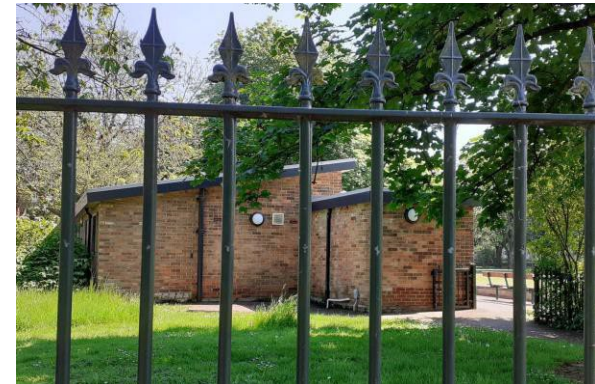
New external lighting at the Bowls Pavilion
