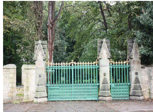
Hull General Cemetery Gates after renovation
