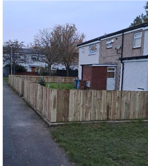
Wenlock st gates and fencing
