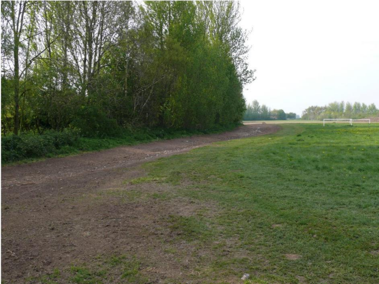
New swale on Howdale Road awaiting seeding
